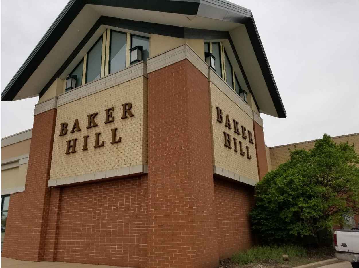
MOUNTED WALL SIGN LOCATED ON THE SOUTH EAST CORNER OF THE BUILDING
