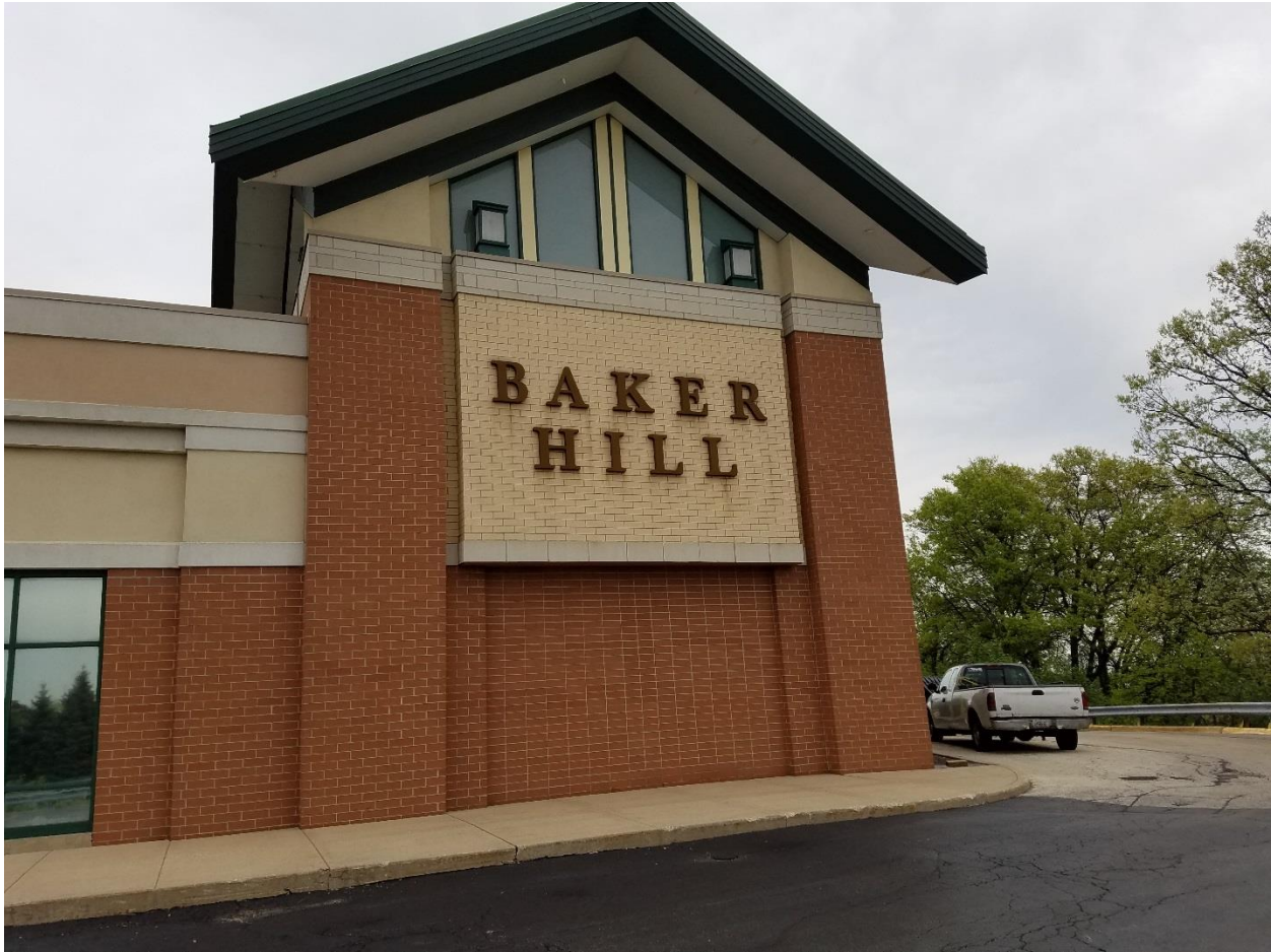
MOUNTED WALL SIGN LOCATED ON THE SOUTH EAST CORNER OF THE BUILDING, SIGN IS ON THE WEST FACING WALL OF THE BUILDING
