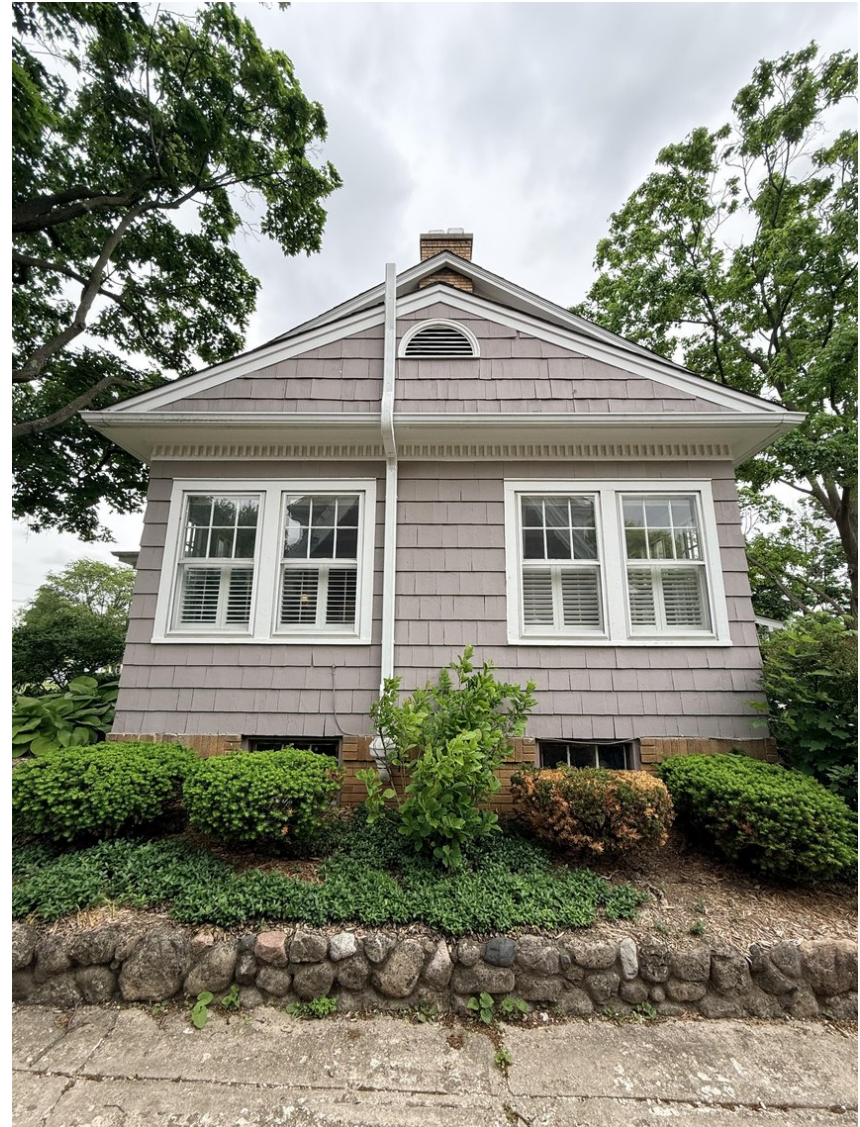
Figure 32: South Elevation, Facing North — Sunroom / Enclosed Porch
