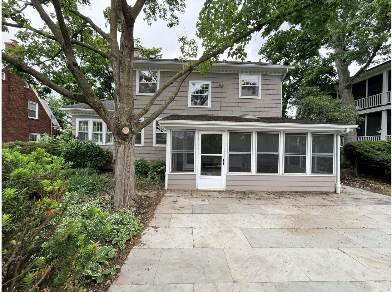
Figure 33: East (Rear) Facade
