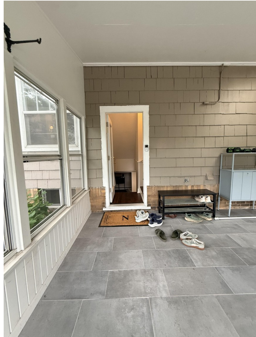
Figure 50: Enclosed Rear Porch, Rear Façade Entrance
