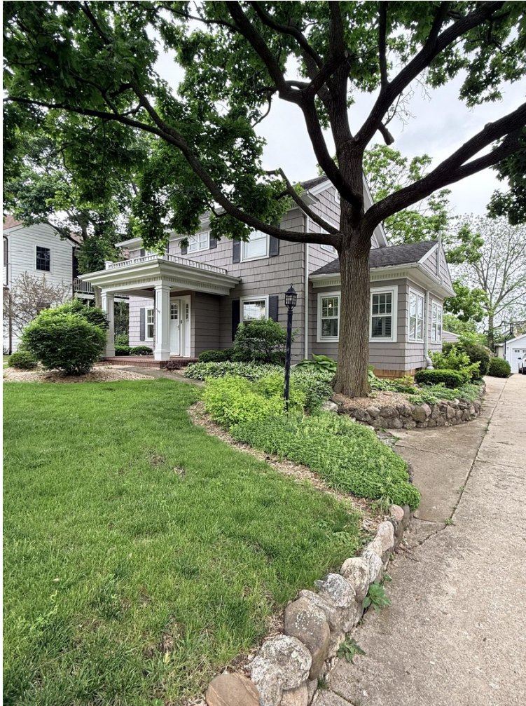
Figure 29: Southwest Corner, Facing Northeast
