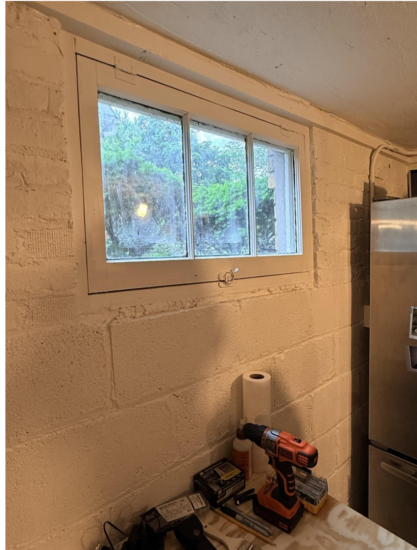
Figure 58: Basement, Window Detail
