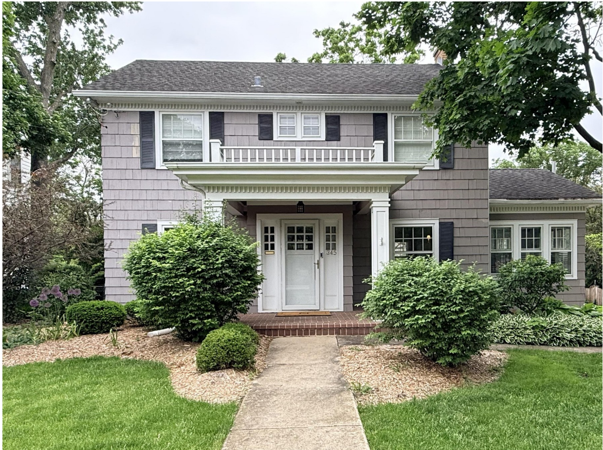
Figure 26: Primary (West) Façade, Facing East
