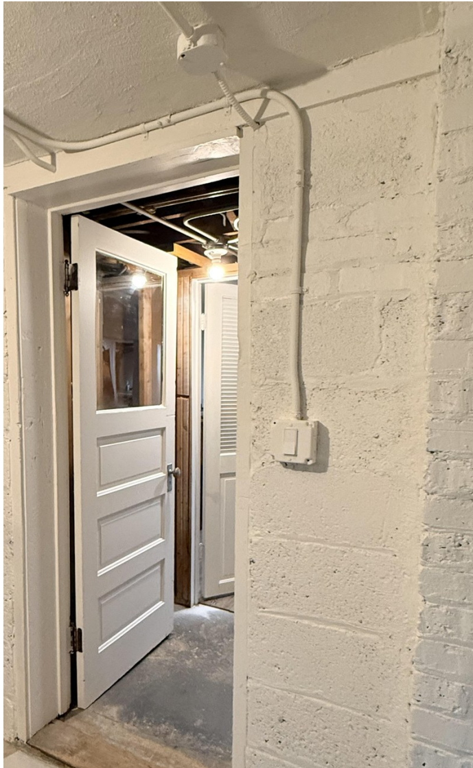
Figure 57: Basement, Unfinished Storage Room
