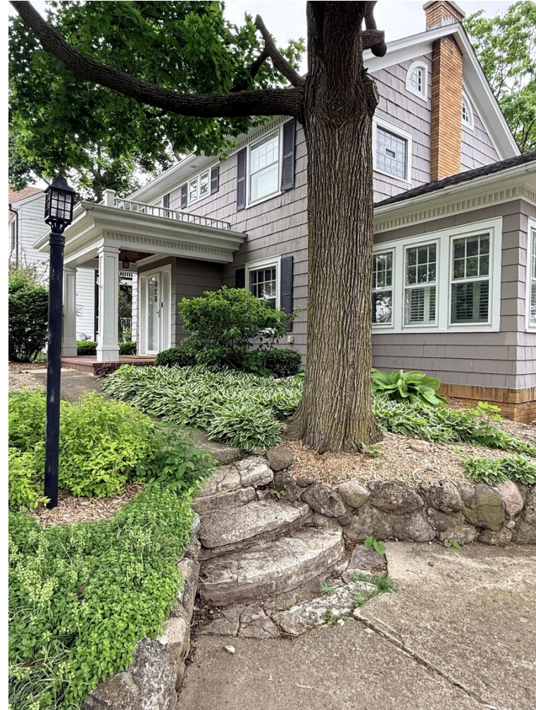
Figure 30: South Elevation, Facing North
