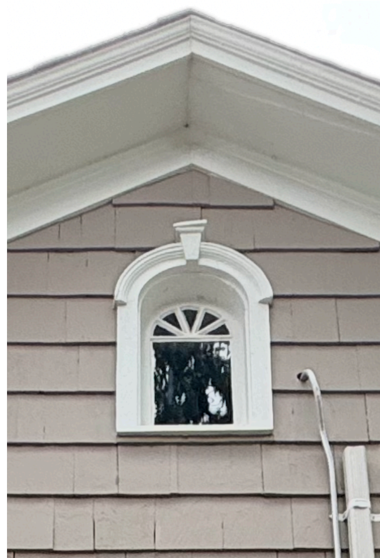
Figure 36: North Facade, Window Detail
