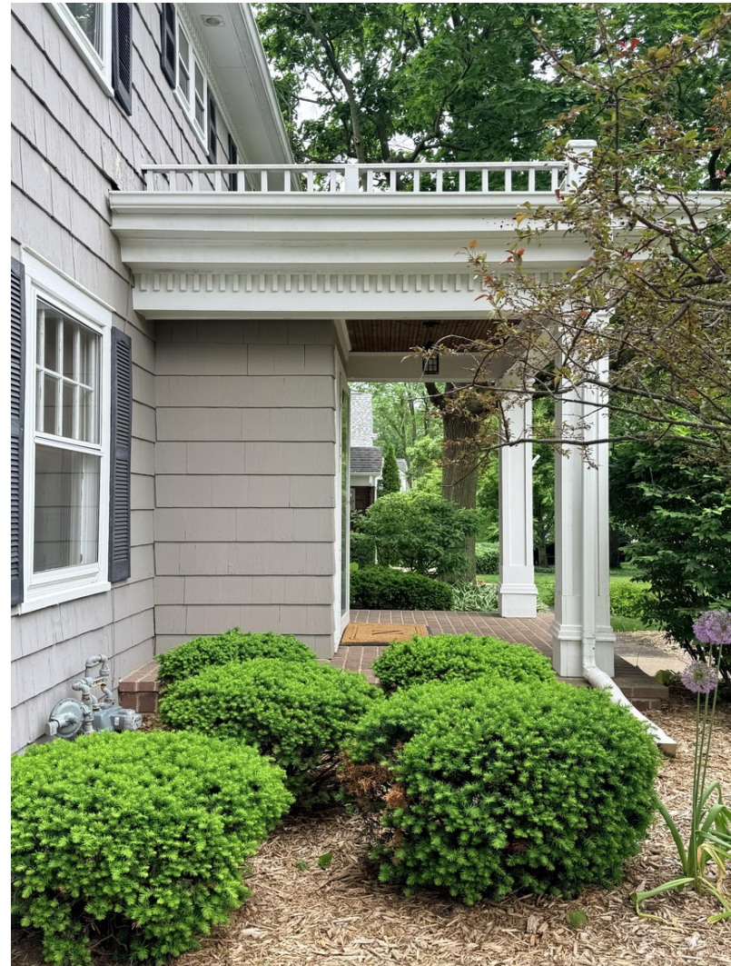
Figure 28: Front Porch, Facing South
