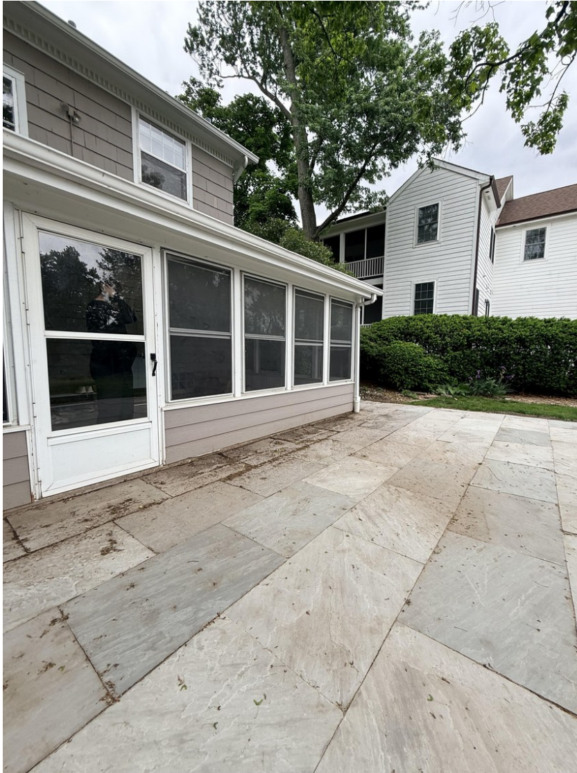
Figure 35: Rear Facade, Detail of porch
