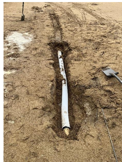
Bunker repair on hole 9 fairway.
