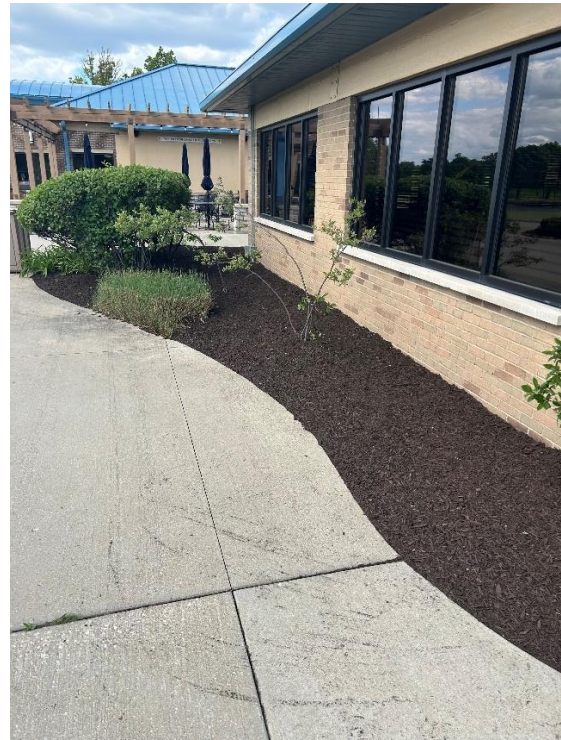
Grounds crews began installing mulch throughout the course, clubhouse area and parking lot.
