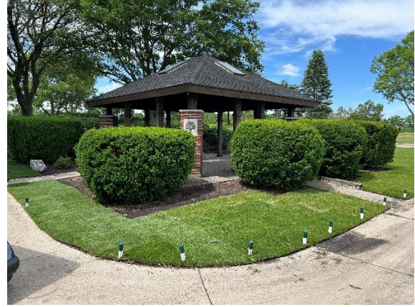
Work has begun to improve the aesthetics of our rain shelters. Crews sodded the area around the shelter on #4 (18-hole).
