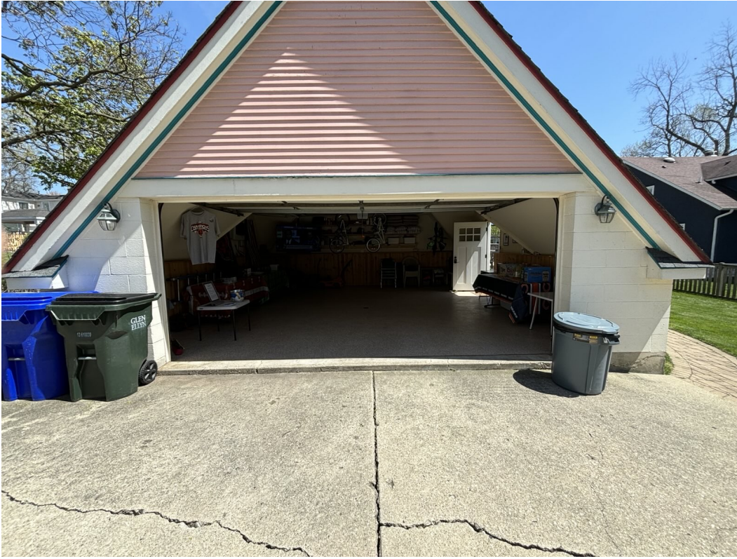
Garage Interior – Full Size
