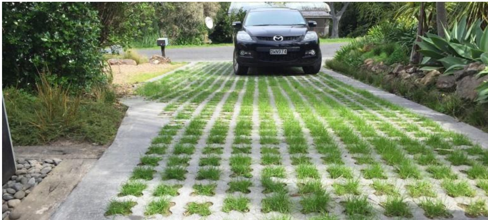
Example of Grasscrete Driveway
