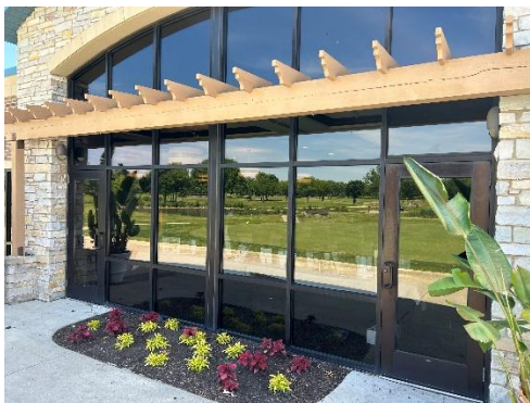
After picture of the wooden pergola located outside of the banquet room.
