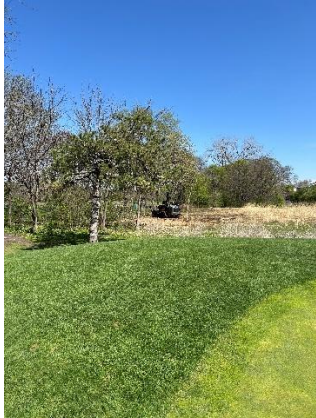
Forestry mulching behind the chipping green between 18 fairway.
