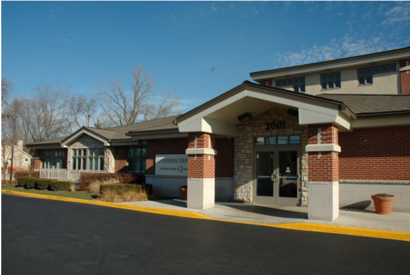
Conerstone Medical Office, NEC Butterfield and Weisbrook Roads – Wheaton
