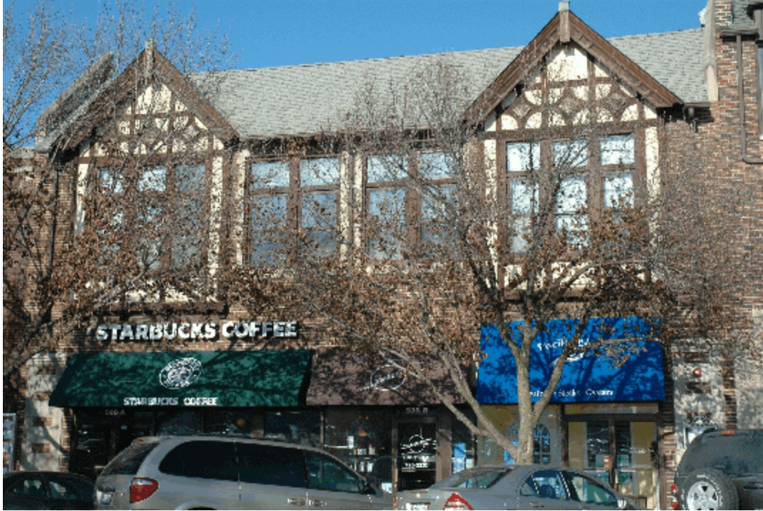
Appropriate Wall Sign Placement, Starbucks – Downtown Glen Ellyn
