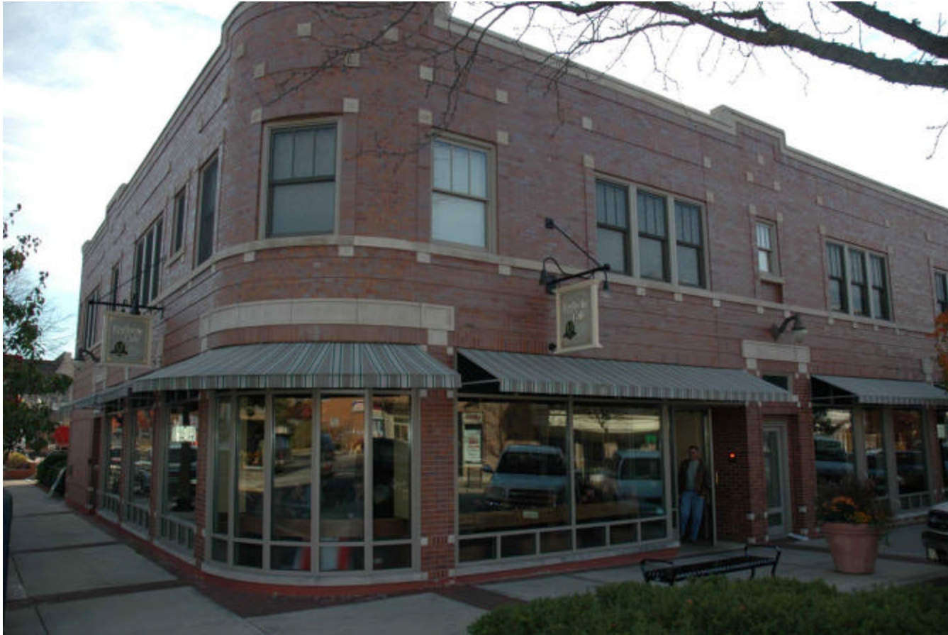
Façade Restoration – Wesley and Hale, Downtown Wheaton
