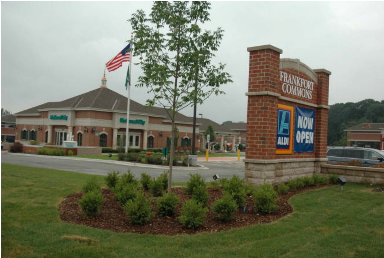
Commercial Center – Frankfort
