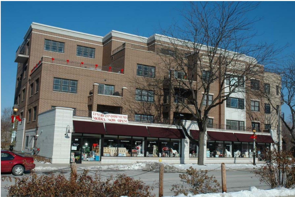
Condominium Development With Ground Floor Retail in the C5B District
