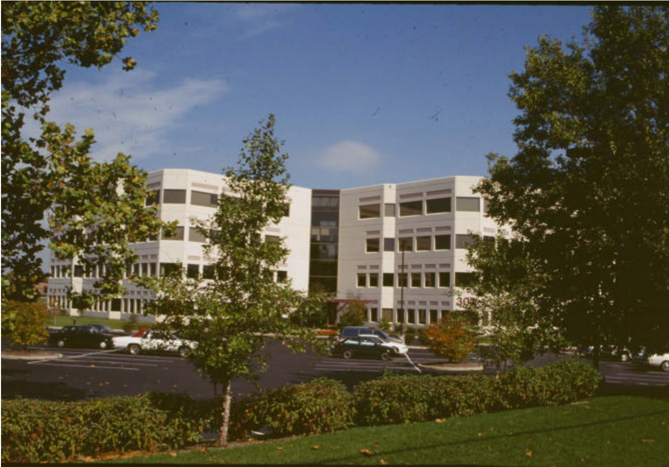
Contemporary Office Building, Army Trail Road – Bloomingdale
