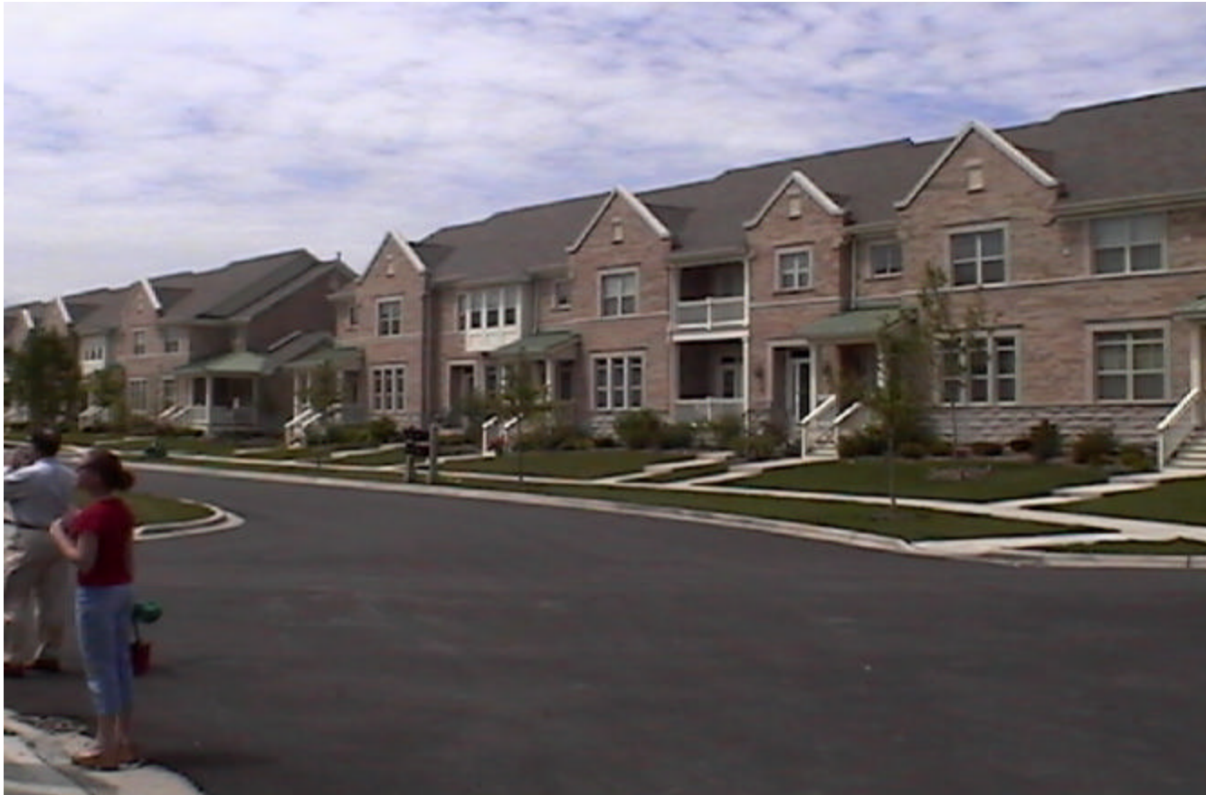
Glenview Naval Air Station Redevelopment – Glenview
