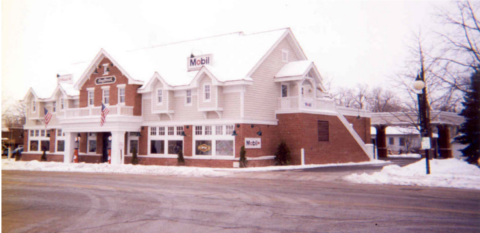
Mobil Gas Station and Commercial Space – Contributed by Lee Marks, GE Historical Commission
