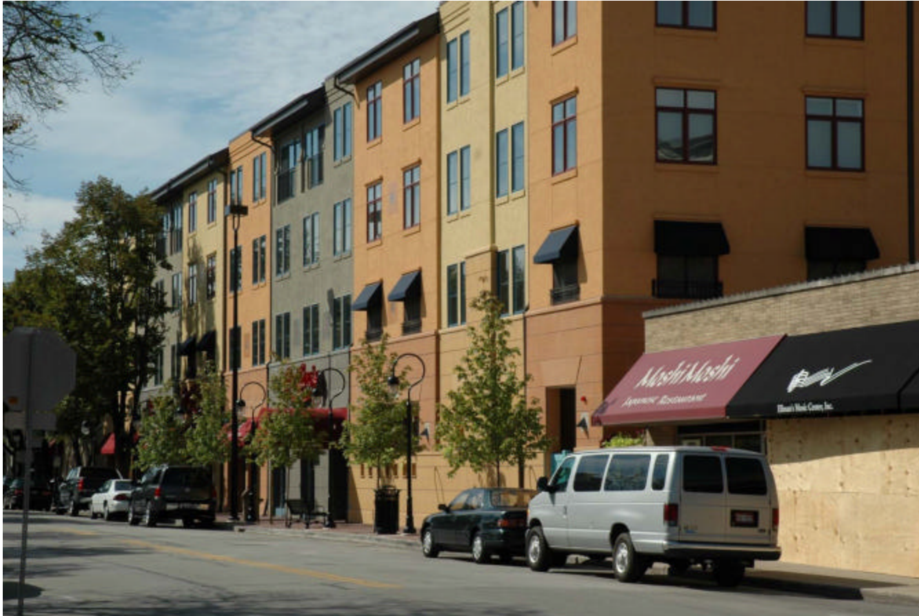
Multi-family Housing – Naperville
