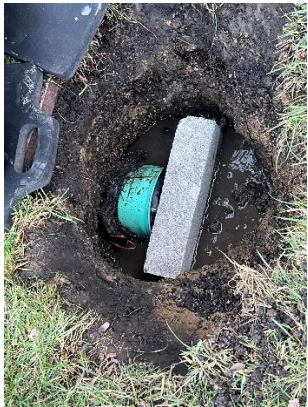
Grounds & maintenance crews repaired several drainage problems throughout the course.
