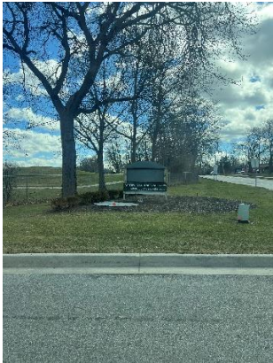
The Reserve 22 sign on Lambert Avenue was damaged.
