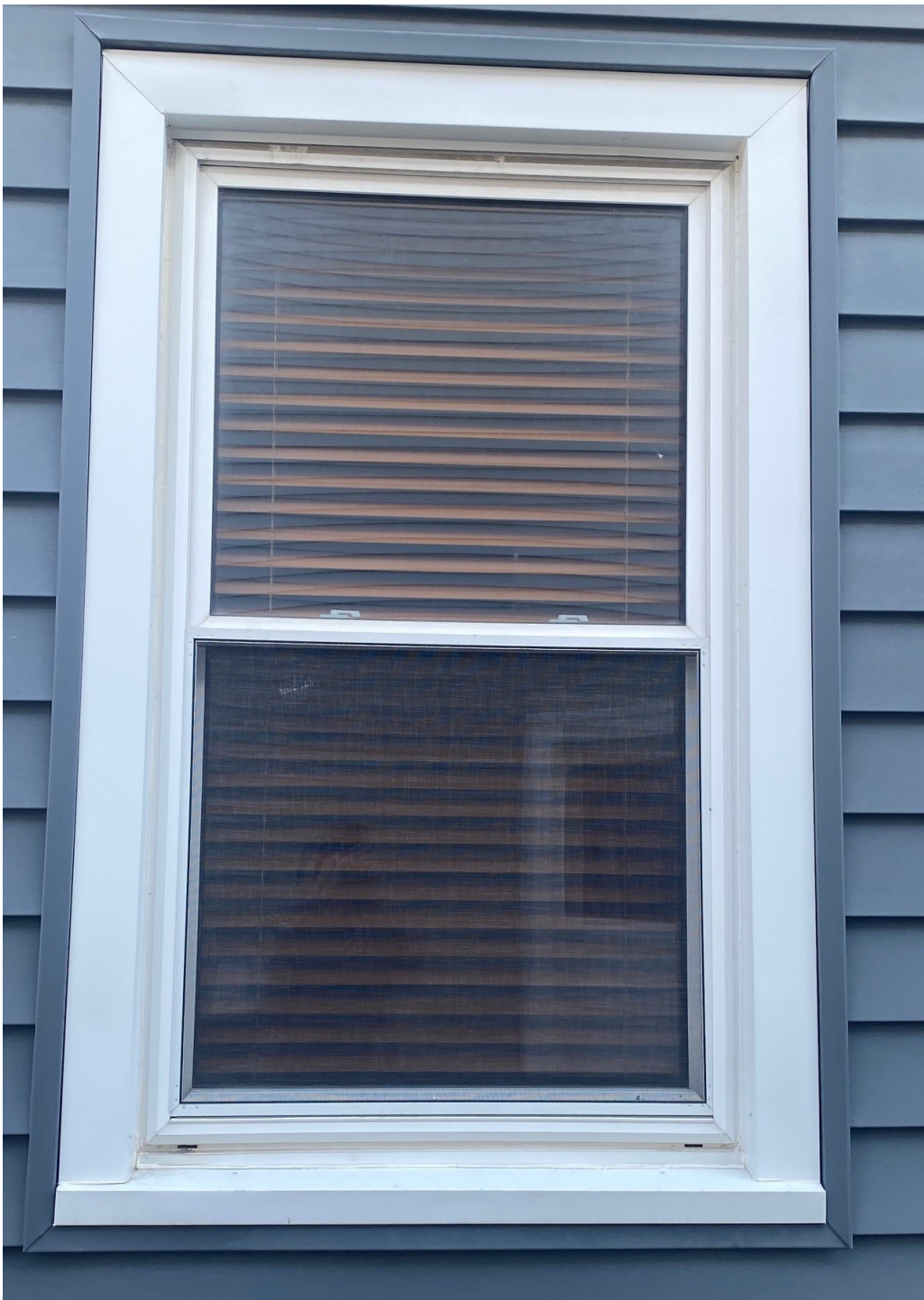
Vinyl Window on the side of the house
