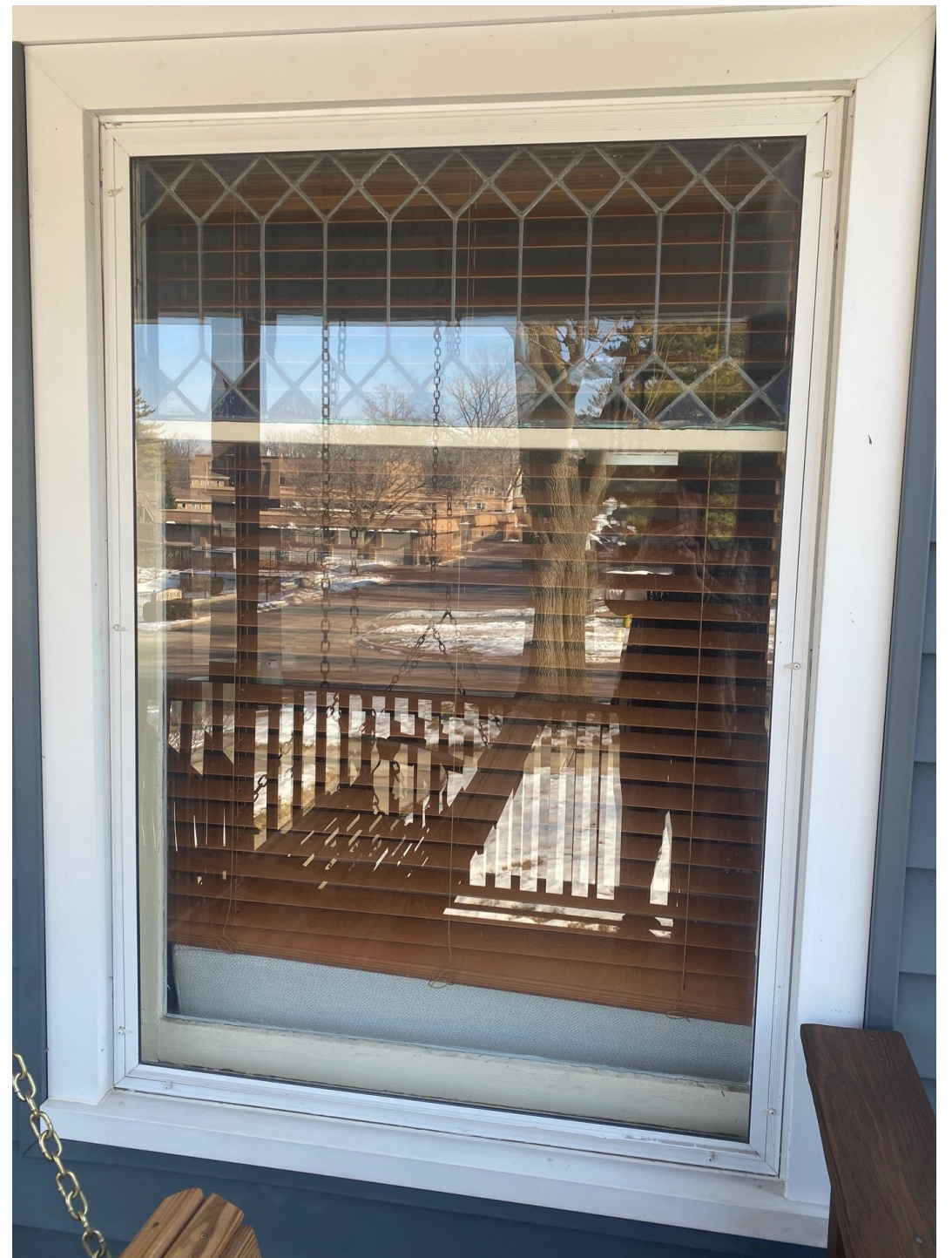
Front single pane picture window with non-original storm window
