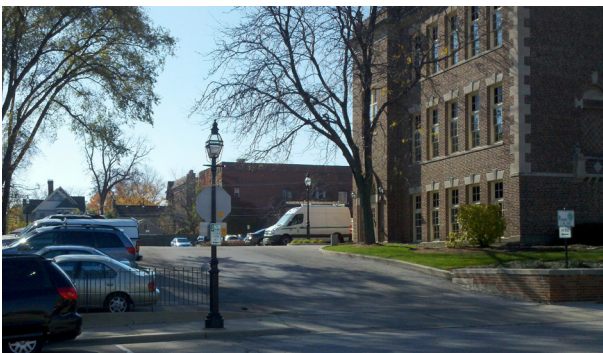
Parking lot entrance ramp too steep: safety hazard
