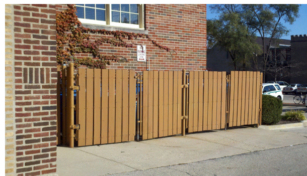
Trash pick-up area conflicts with sally port entrance
