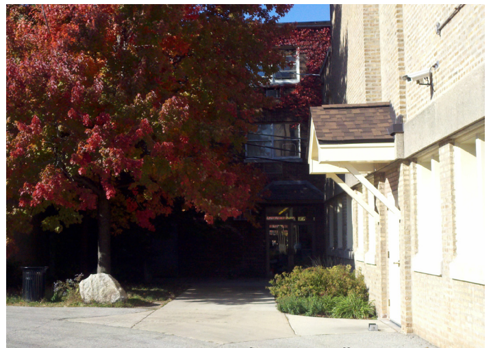
Hardware store delivery lane conflicts with staff entrance
