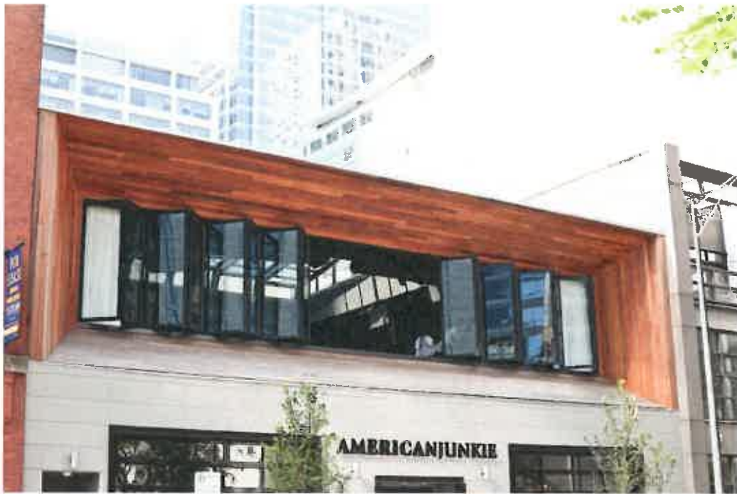
Restaurant American Junkie - River North, Chicago IL - 50' Span
