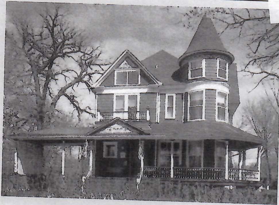
Lawrence C. Cooper Home 545 Park Boulevard Built in 1893, Plaqued by GEHS in 1973
