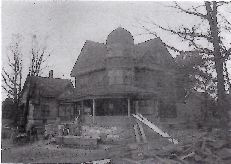
Ward B. LeStage Home, 570 Anthony (Under Construction)
