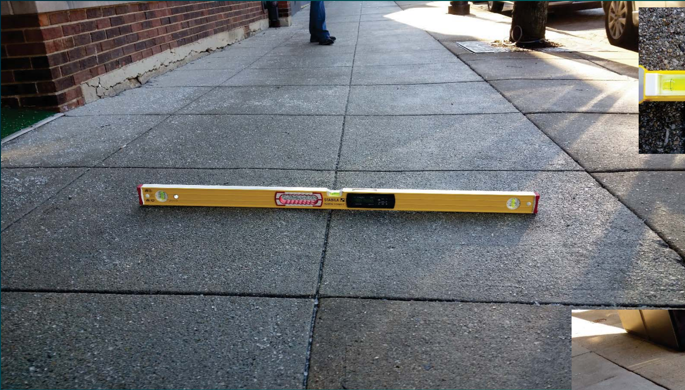
Excessive sidewalk cross slope
