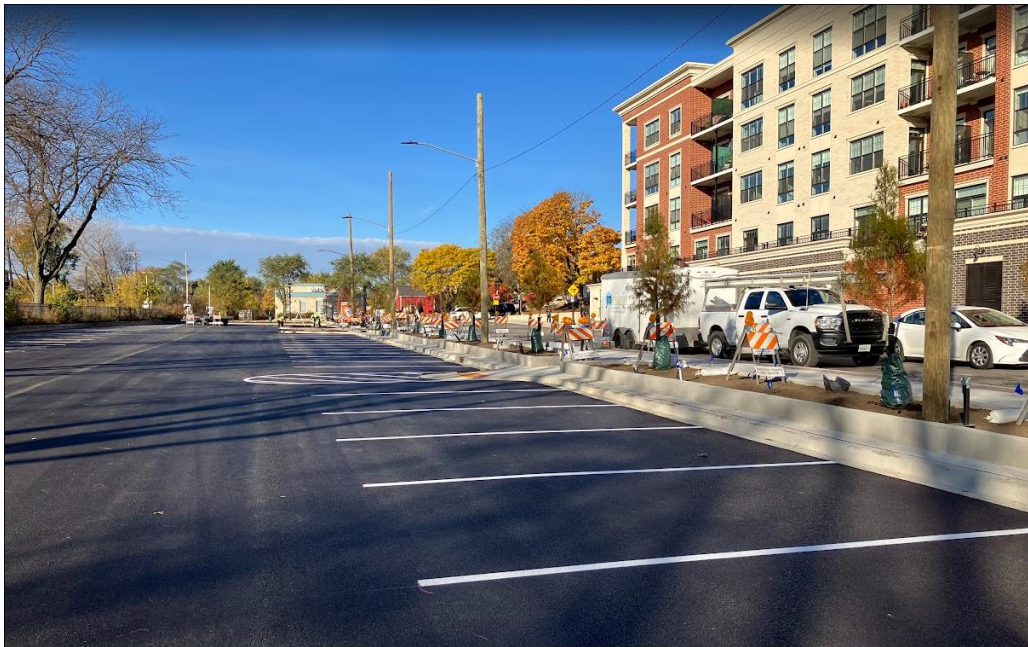
Parking lot just after resurfacing and application of new pavement markings
