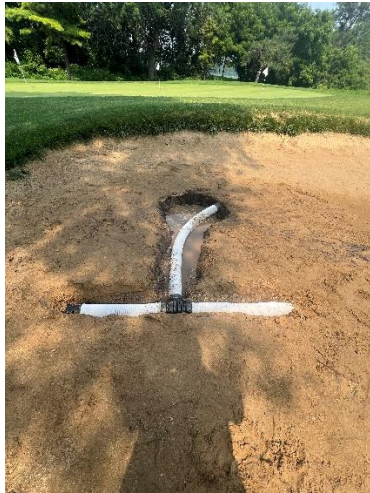
Drainage repair on our practice bunker.
