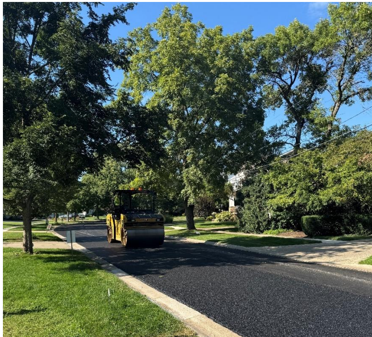
Asphalt Surface Paving on May Avenue 9/4/2025
