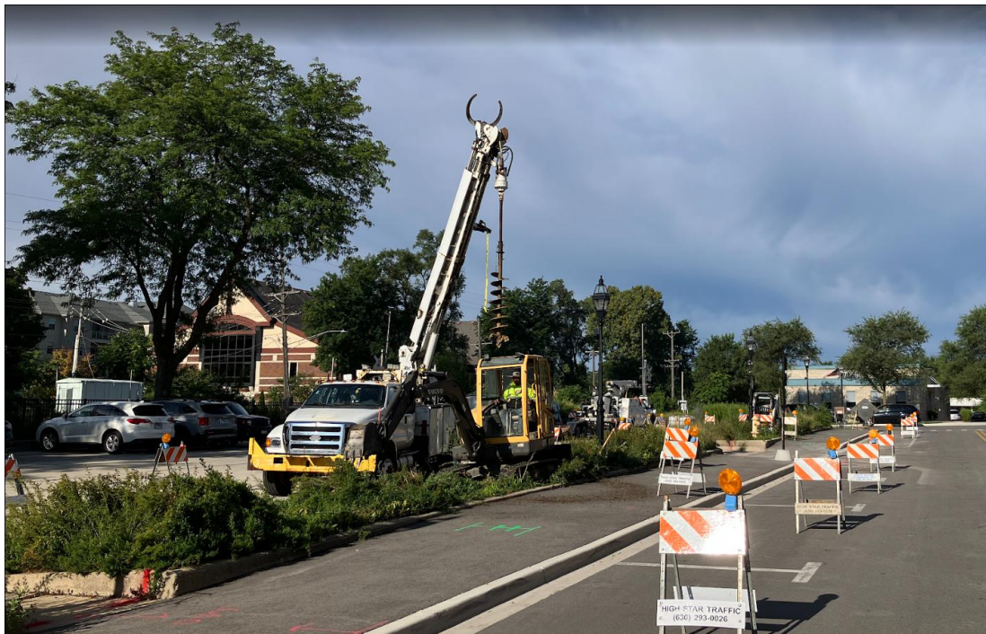
Augering for Temporary Wood Light Pole at the Crescent-Glenwood Lot
