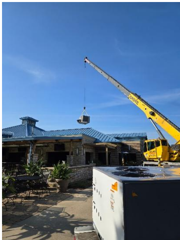
A crane removes our old rooftop AC unit.
