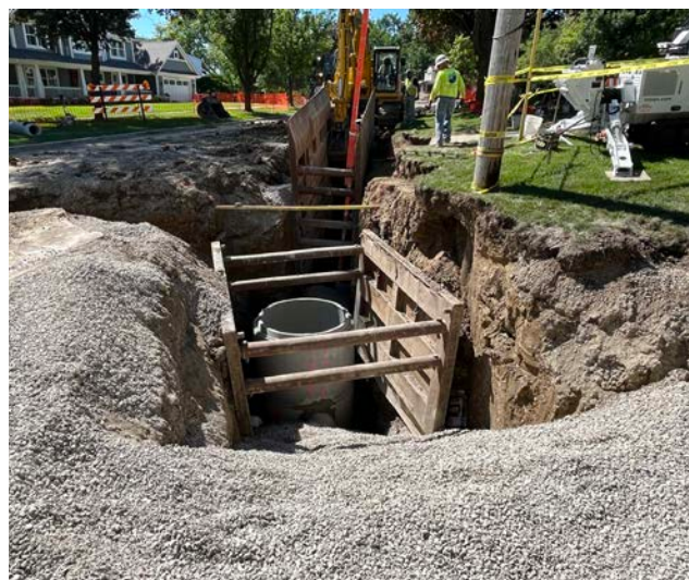
V3's constructability review for the 2022 Residential Roadway & Utility Improvements project identified and avoided potential conflicts with sanitary sewer to keep the project on track.
