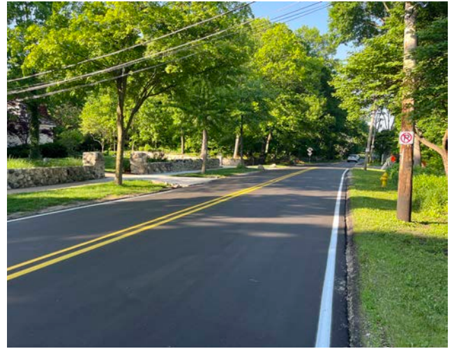
Detailed coordination with residents and utility company, ComEd, resulted in minimizing impacts to both trees and schedule.
