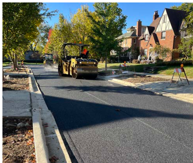
The 2024 Residential Roadway & Utility Improvements project required significant coordination with impacted residents.
