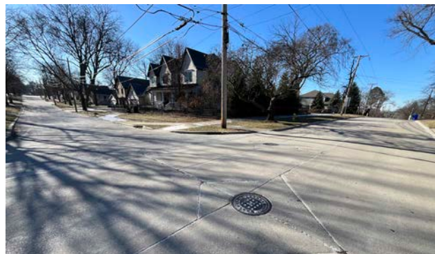
Hill Avenue at Travers Avenue Intersection. Sanitary sewer replacement to structure S-583 (pictured above) will require concrete pavement patching and extended detour that are not accounted for in the provided plan set.
