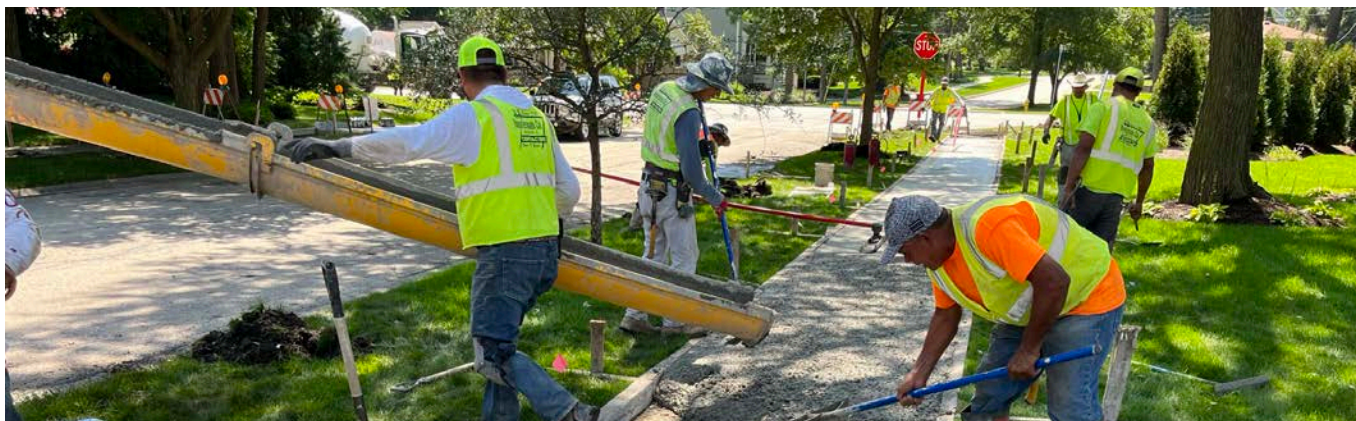
More than 700 residences were located within the 2023 Residential Roadway & Utility Improvements project limits. V3 hand-delivered project notifications to each residence regarding construction.
