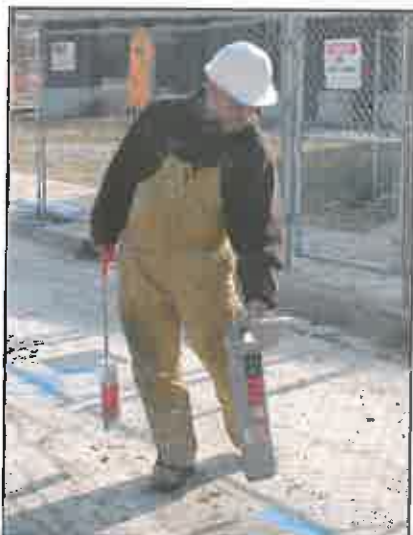
"Critical Dig" Location Specialists
