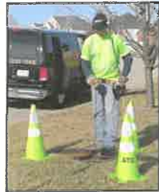
Ultrasonic Leak Detection
