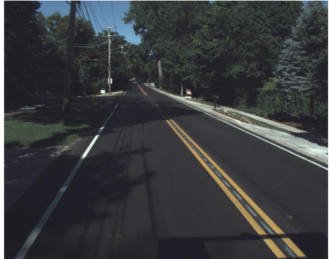
CRESCENT DRIVE – Section 249 Crescent Blvd to End PCI 100
