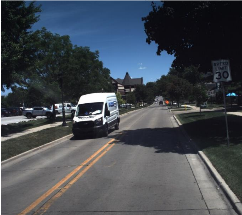
DUANE ST – Section 680 Lorraine St to Melrose Ave PCI 83
