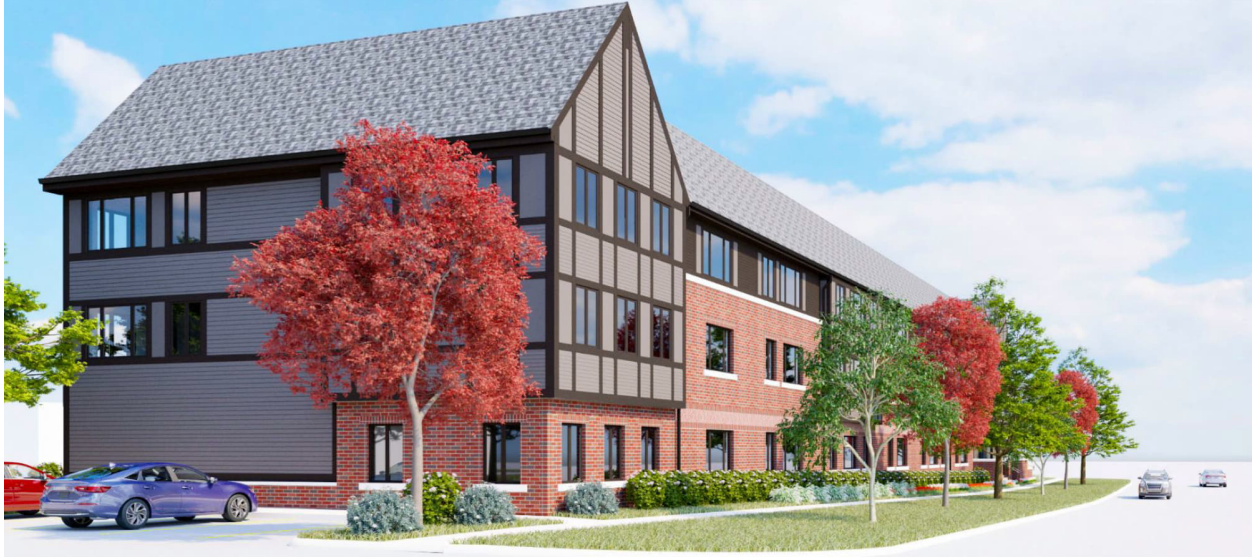
West Façade looking Northeast
