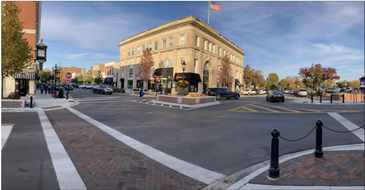
Completed crosswalk at the Crescent/Main intersection
