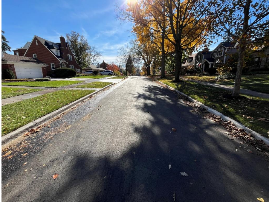
2024 Utility and Roadway Improvements Crest Road
