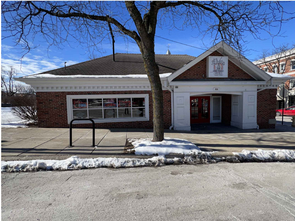
VIEW FROM MAIN STREET SIDE OF BUILDING
