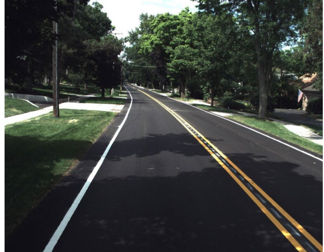
APPIAN WAY – Section 671 Forest Ave to End PCI 100
