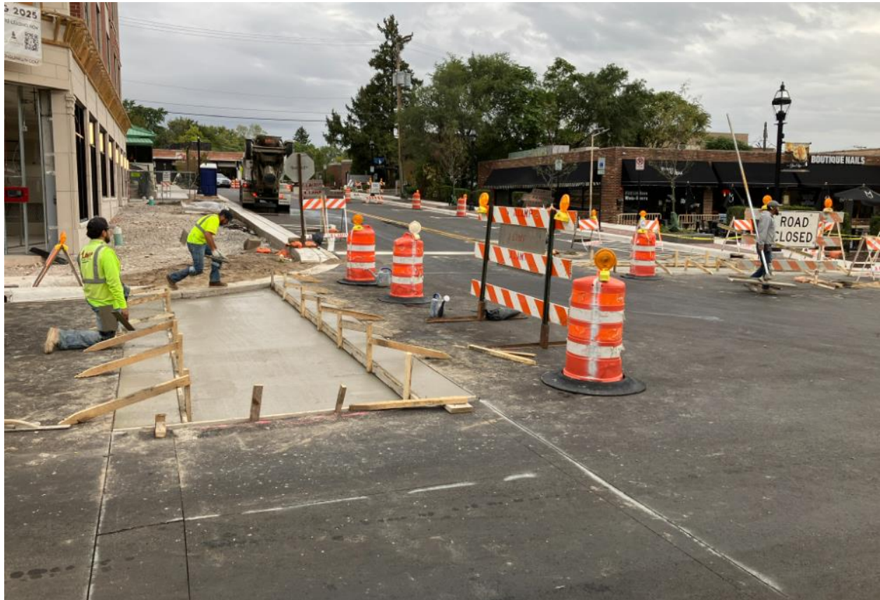
Finishing of the concrete pour for the brick paver crosswalks at Crescent/Glenwood
