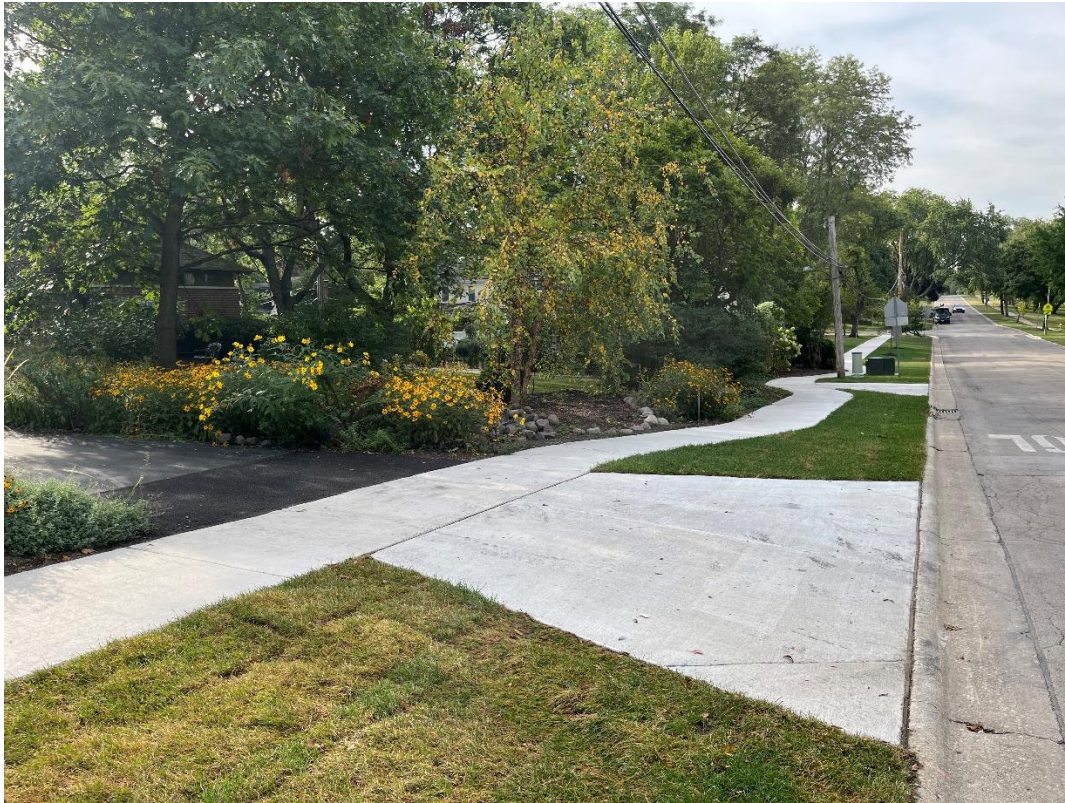
New Sidewalk Installation on Brandon Avenue between Fairview Avenue & Greenfield Avenue
