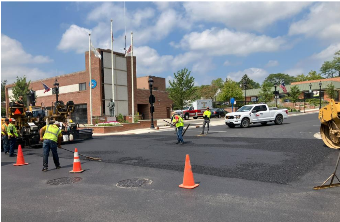
Final asphalt surface being placed within the Main Street/Pennsylvania Avenue intersection
