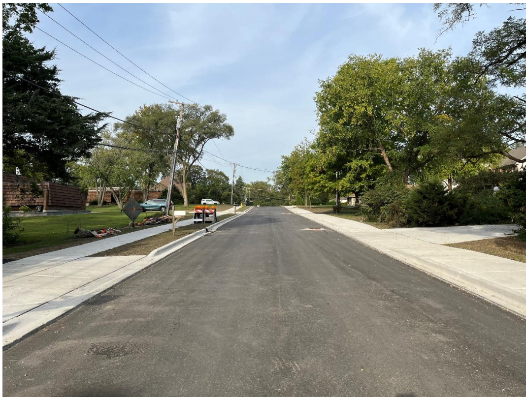
Bemis Road after asphalt binder paving and topsoil spreading
