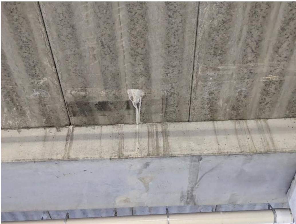
Photo 34. Water leakage and efflorescence from underneath a hollow core void.
