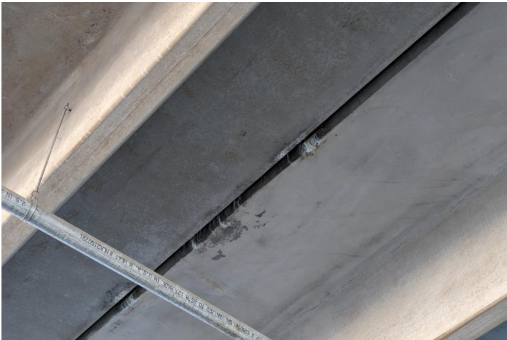
Photo 32. Typical water leakage and efflorescence at midspan shear connector in the finger.
