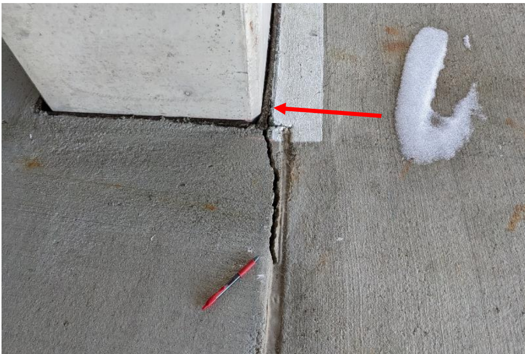
Photo 56. A wide crack that has stemmed off the corner of the column to the construction joint. Also note that the column perimeter is not sealed.
