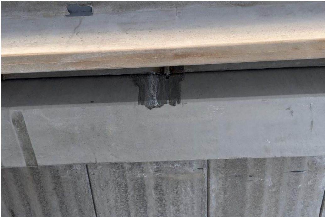
Photo 30. Heavy water leakage at the beam to the finger observed from the 1 st level.
