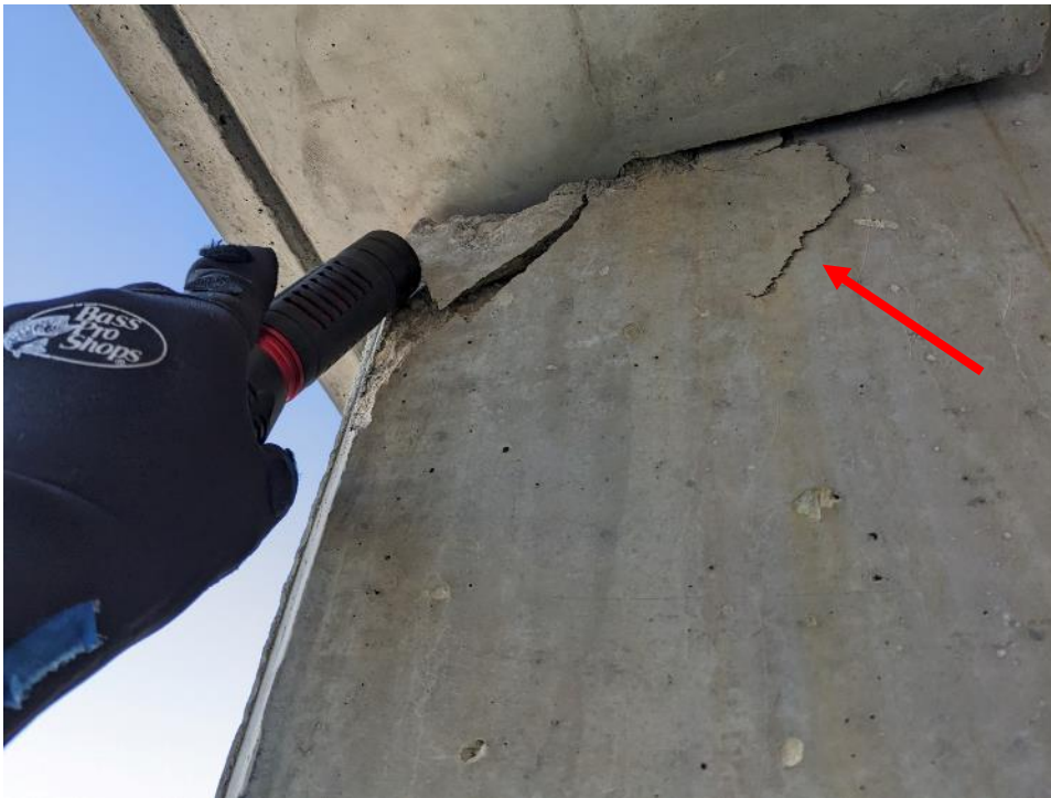
Photo 72. An isolated concrete column delamination on the interior surface.
