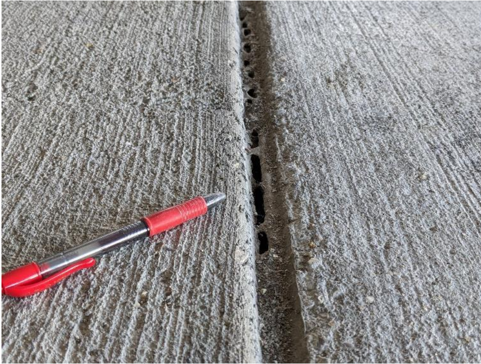
Photo 60. Additional failed construction joint sealant.
