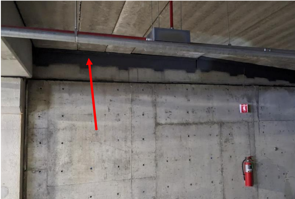
Photo 46. Minimal hollow core bearing at one location supporting the 2 nd level ramp.
