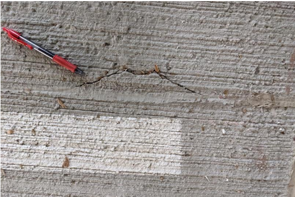
Photo 48. Isolated concrete delamination in the 2 nd level topping slab.
