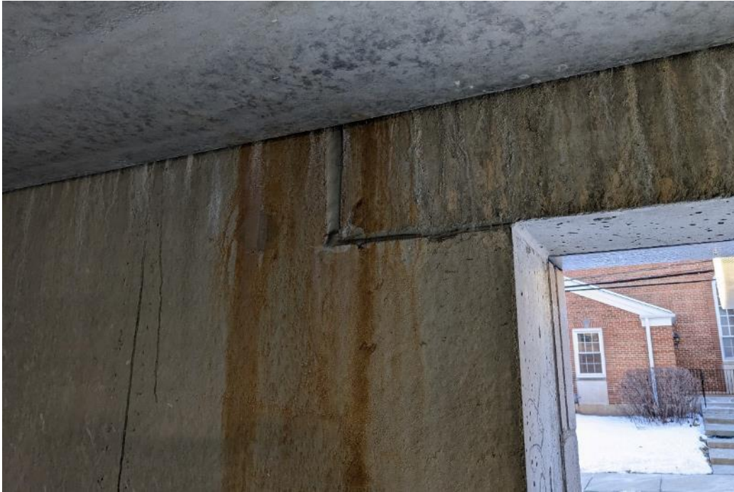
Photo 30. Heavy water leakage at the beam to the finger observed from the 1 st level.
