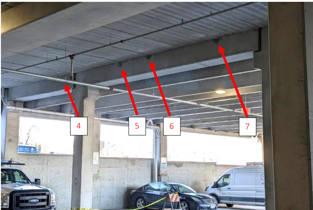
Photo 8. Overall view of concrete spalls at the inverted tee beam at Grid 7.8, separating the main structure from the finger.
