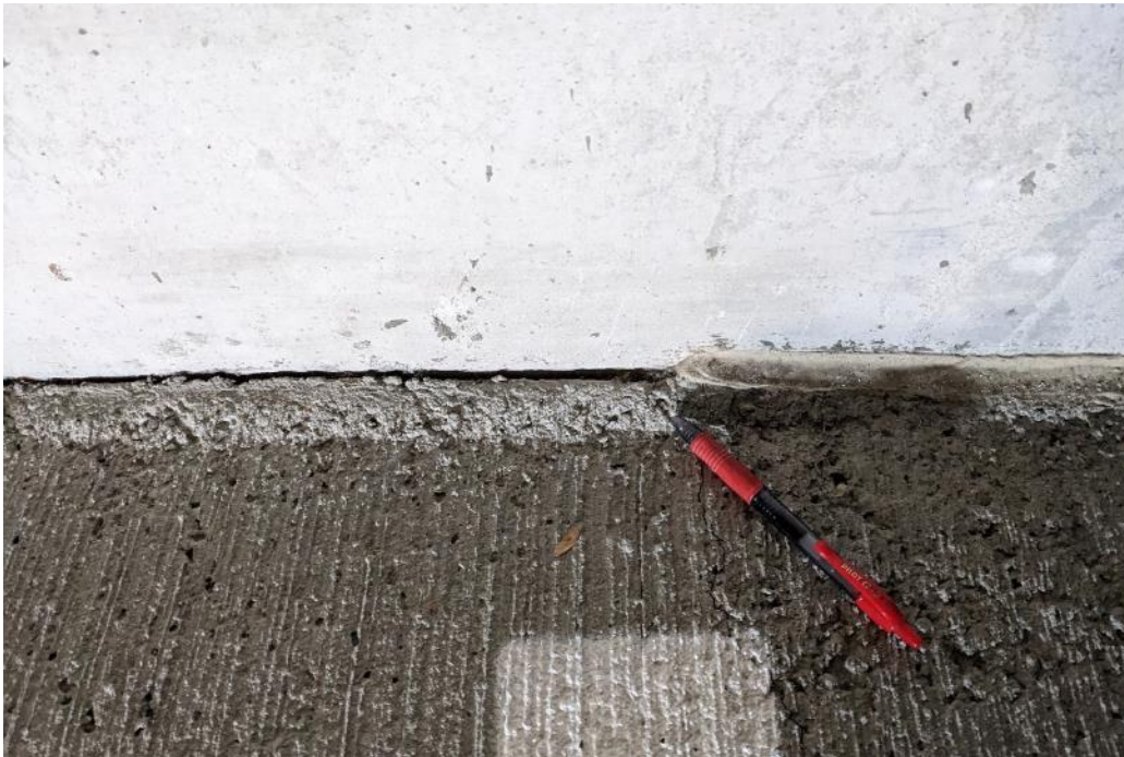
Photo 62. Cove sealant at the wall bases was typically missing at areas except at limited areas at the south end.
