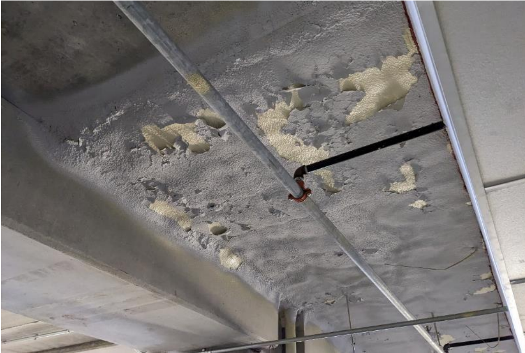
Photo 48. Isolated concrete delamination in the 2 nd level topping slab.
