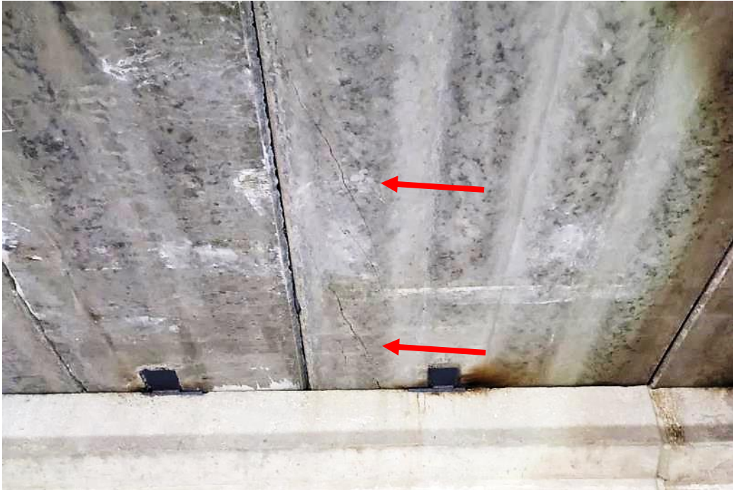
Photo 40. Another crack on a hollow core plank with efflorescence.
