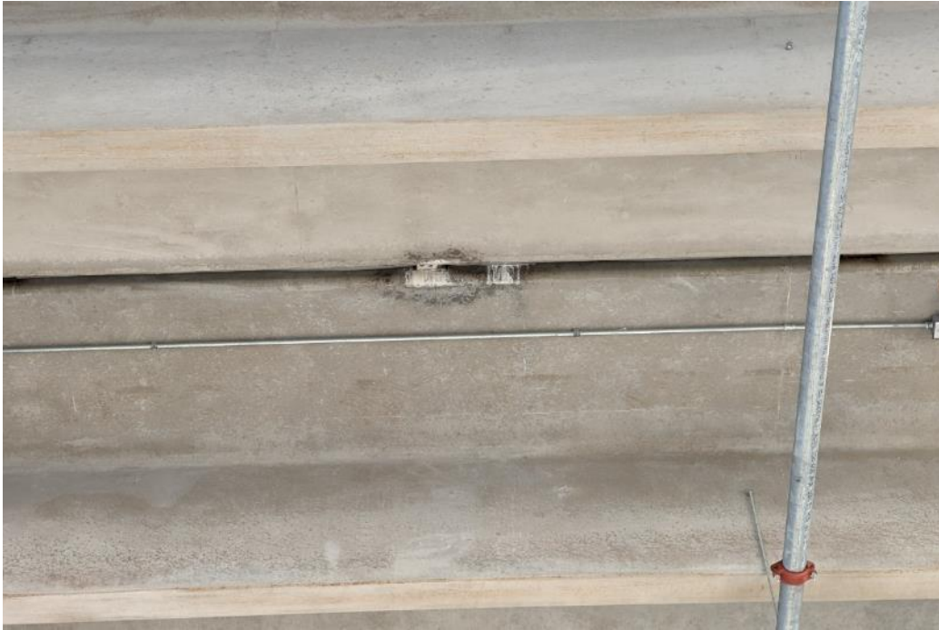
Photo 32. Typical water leakage and efflorescence at midspan shear connector in the finger.
