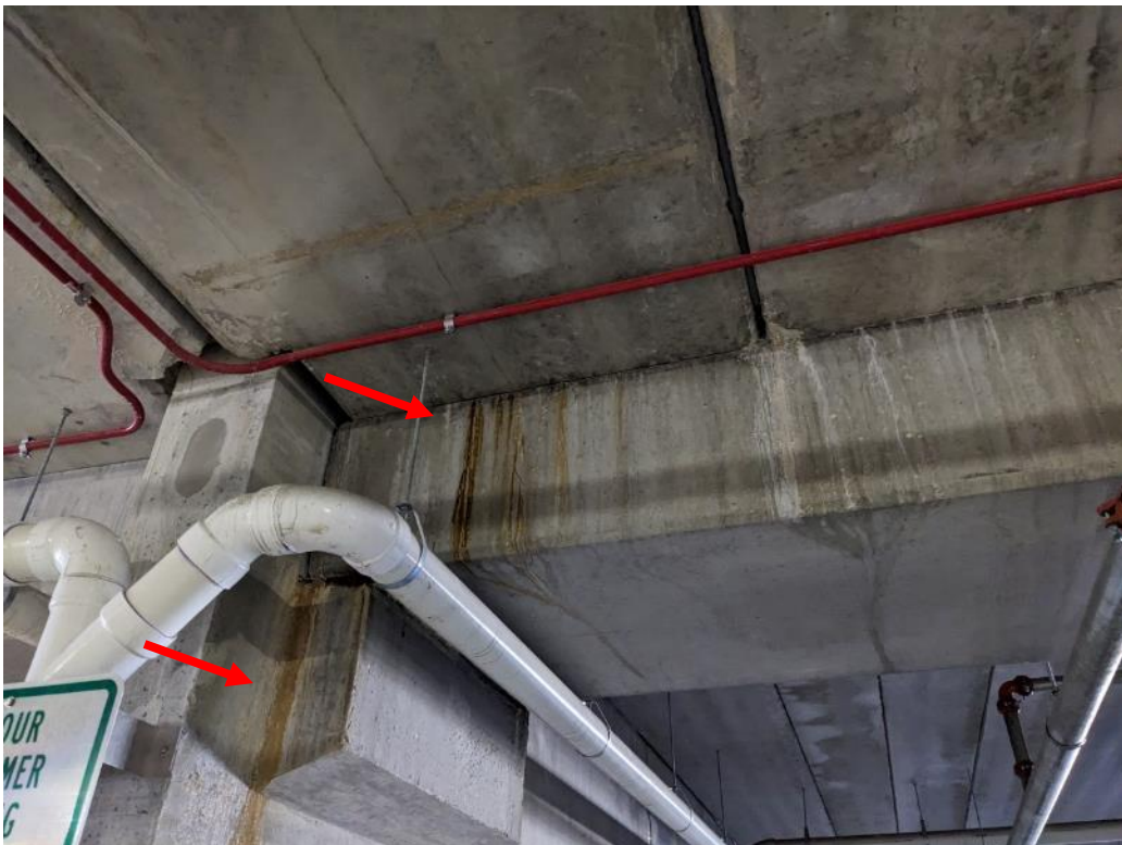
Photo 28. Water leaching and corrosion stains along the length of a beam observed from the 1 st level.
