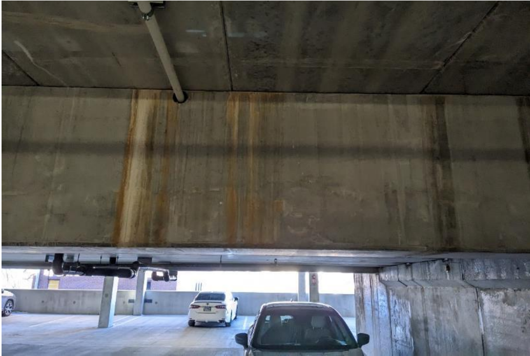
Photo 70. Active leaking observed on underside of 3 rd level hollow core void into the parking area.
