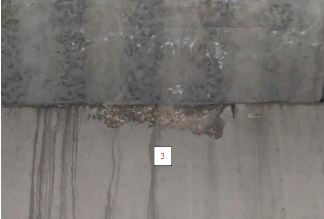
Photo 8. Overall view of concrete spalls at the inverted tee beam at Grid 7.8, separating the main structure from the finger.
