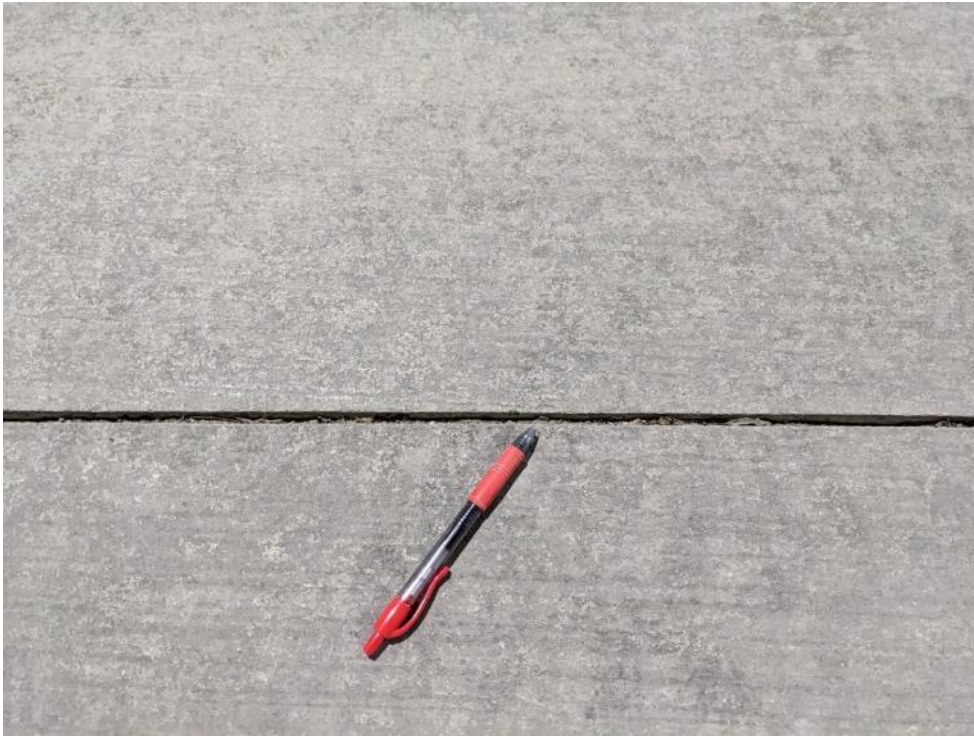
Photo 18. Typical slab-on-ground with missing control joint sealant.
