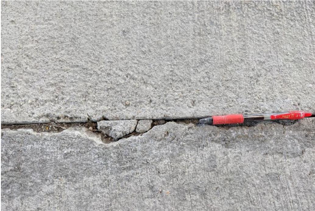
Photo 20. Missing slab-on-ground control joint sealant with small spalls along the joint in the finger.
