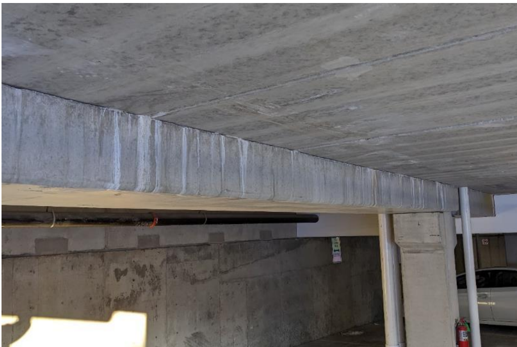
Photo 26. Water leaching stains typical along the length of a beam observed from the 1 st level.
