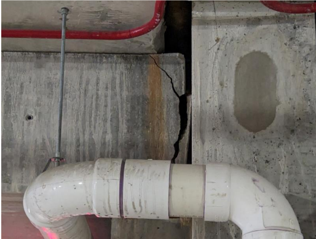
Photo 42. A small delamination of a beam haunch between hollow core planks along Grid Line 1.
