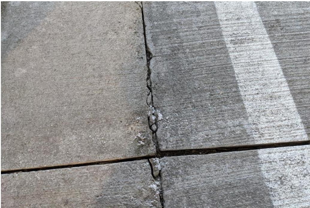
Photo 20. Missing slab-on-ground control joint sealant with small spalls along the joint in the finger.
