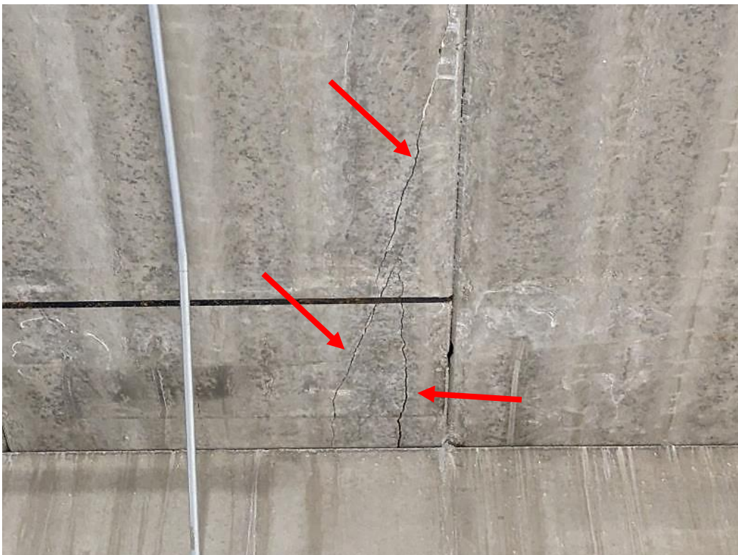
Photo 36. Close-up of the hollow core crack from the previous photo.
