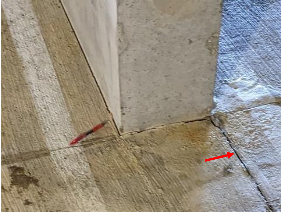
Photo 64. Cove sealant was typically missing at the column bases.
