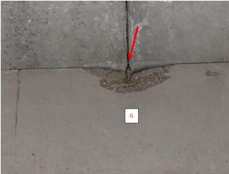
Photo 12. Spall 7 along Grid 7.8 from Photo 8. Note, presence of dowel at center of spall.
