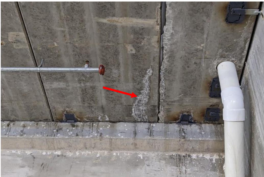
Photo 40. Another crack on a hollow core plank with efflorescence.
