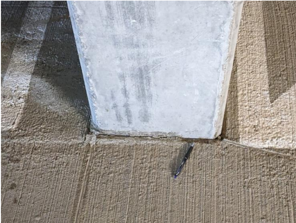
Photo 64. Cove sealant was typically missing at the column bases.
