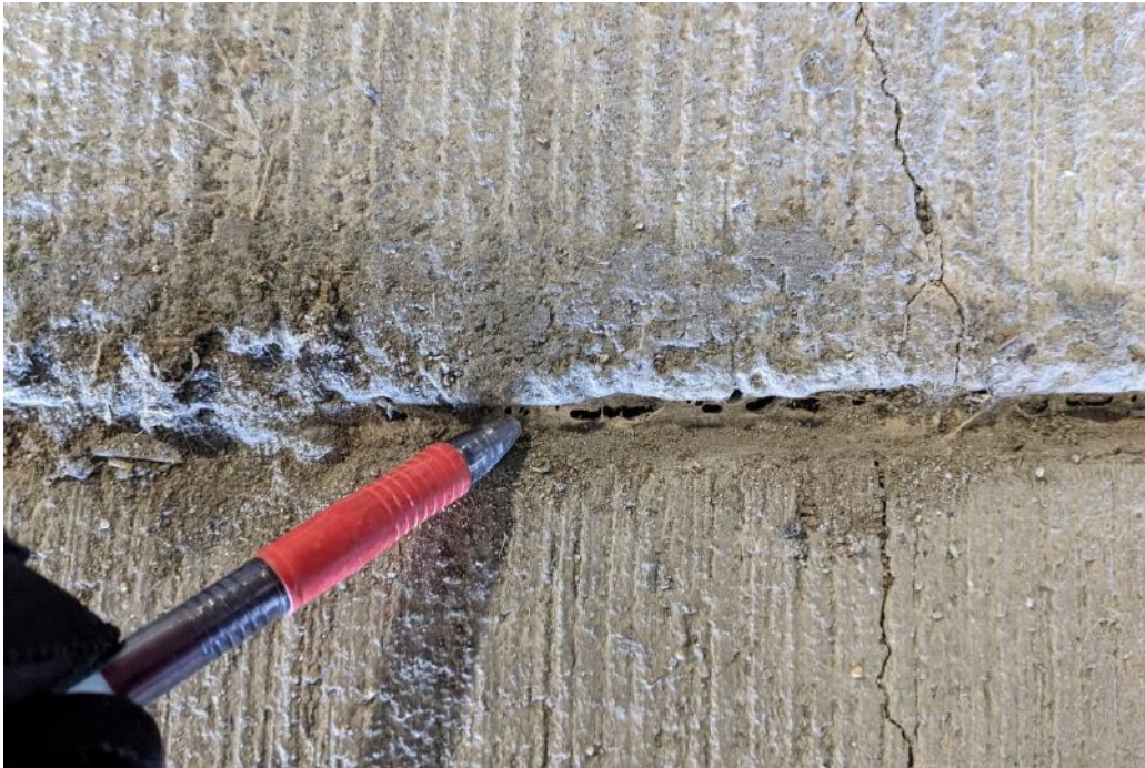
Photo 60. Additional failed construction joint sealant.
