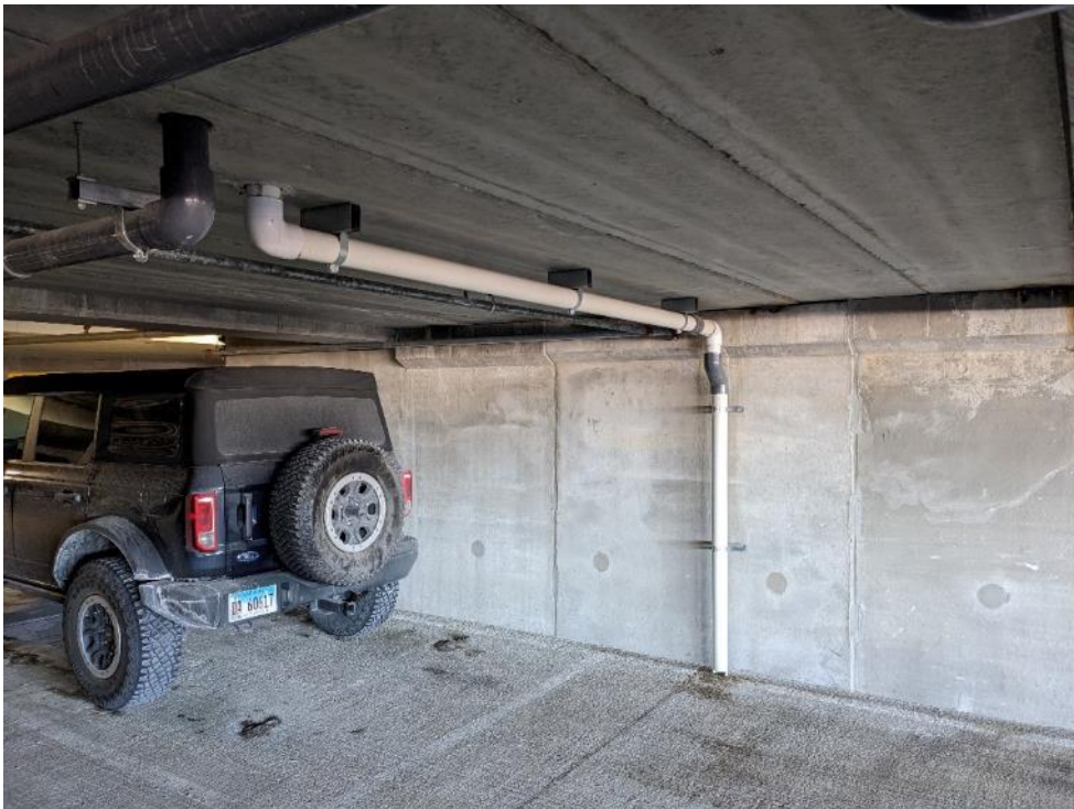
Photo 74. Plaza level drainpipe draining directly onto 2 nd level floor.
