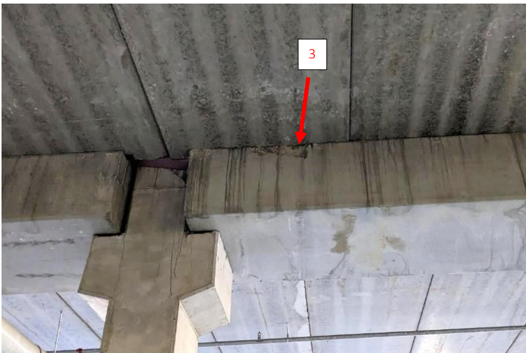
Photo 6. Concrete spall in inverted tee beam at Gridline 5.
