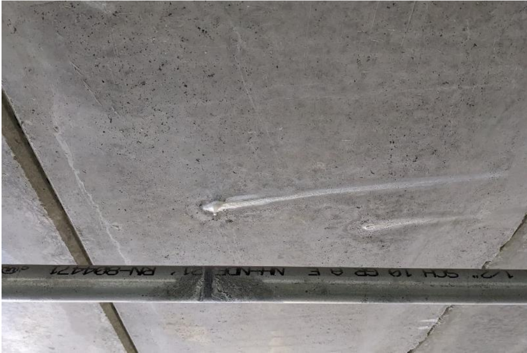
Photo 34. Water leakage and efflorescence from underneath a hollow core void.
