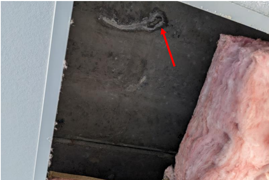
Photo 70. Active leaking observed on underside of 3 rd level hollow core void into the parking area.
