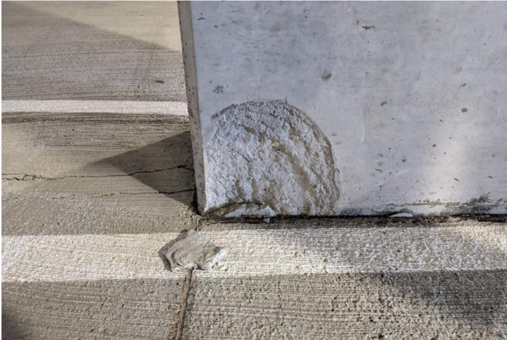
Photo 72. An isolated concrete column delamination on the interior surface.
