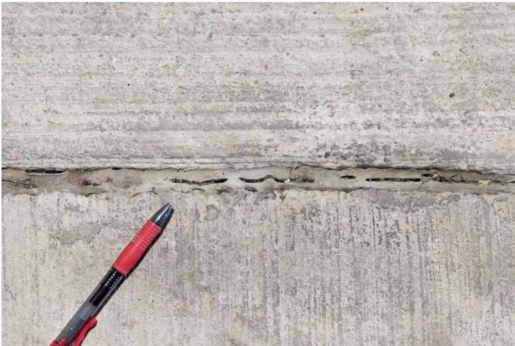
Photo 58. Close-up of failed construction joint sealant from the previous photo.
