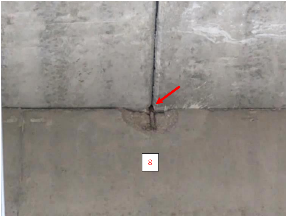
Photo 14. Close-up of Spall 8 along Grid 7.8 from Photo 8. Note, presence of dowel at center of spall.
