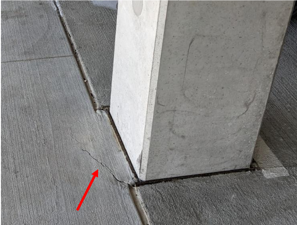
Photo 50. Overall view of a wide crack that extends from wall to column to shear wall.
