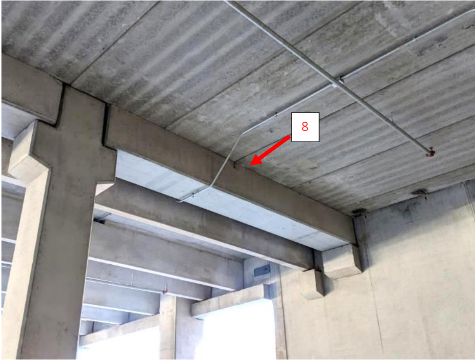
Photo 14. Close-up of Spall 8 along Grid 7.8 from Photo 8. Note, presence of dowel at center of spall.
