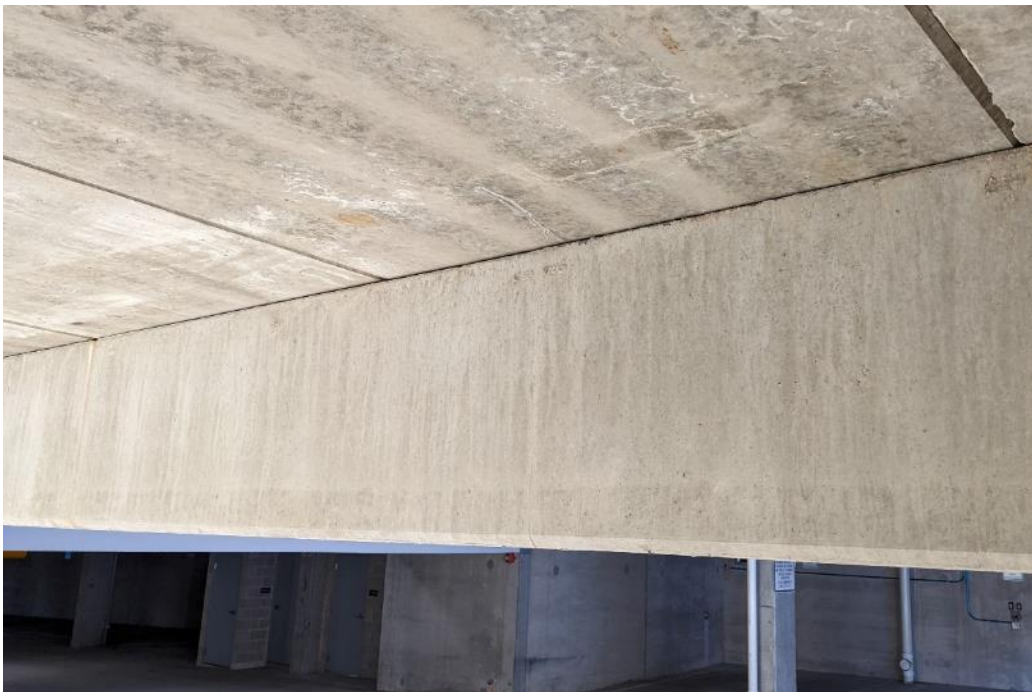
Photo 44. Typical minimal gap separating the hollow core planks from the beams.
