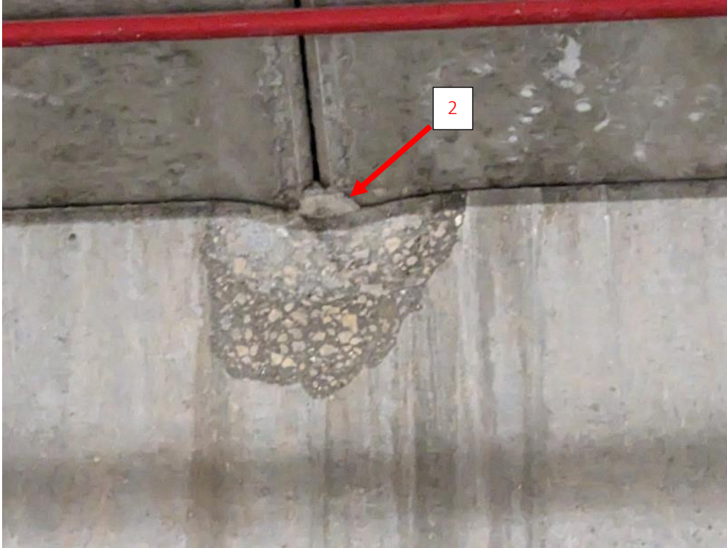
Photo 6. Concrete spall in inverted tee beam at Gridline 5.
