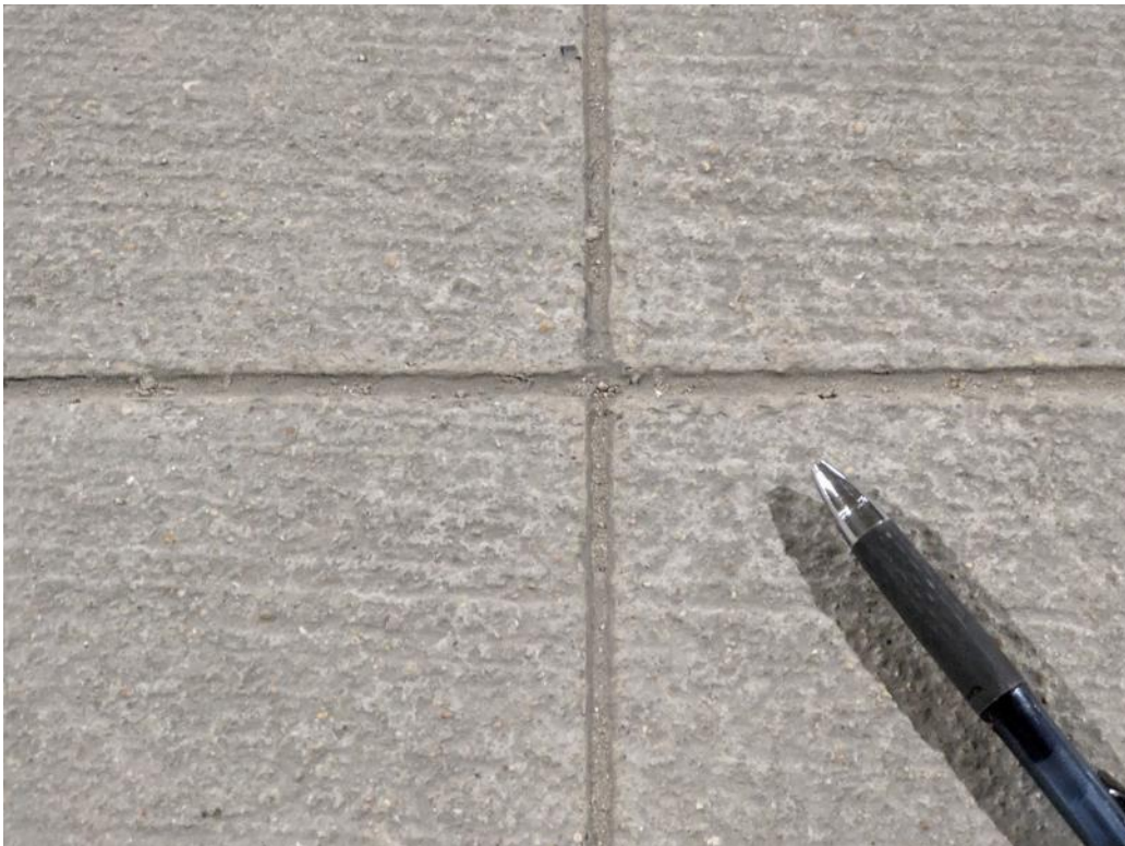
Photo 16. Sealant present in some of the slab-on-ground control joints, typically near the south end.
