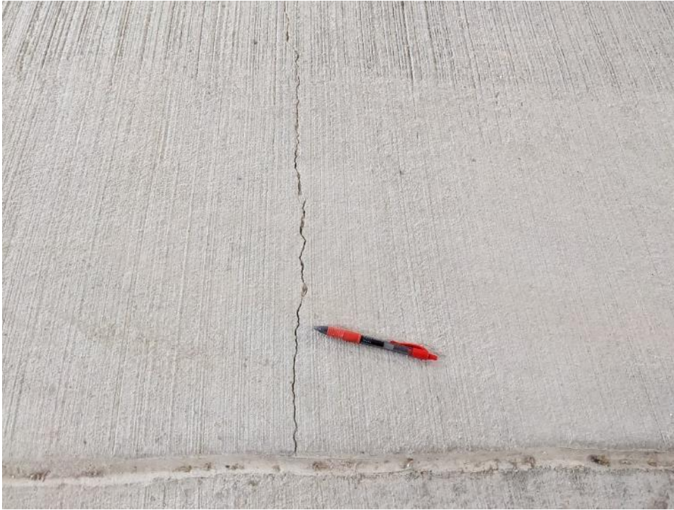
Photo 54. Typical crack in 2 nd level floor topping slab perpendicular to the hollow core planks.
