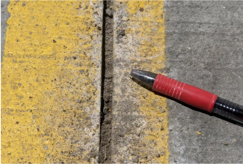
Photo 18. Typical slab-on-ground with missing control joint sealant.
