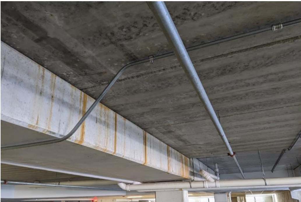
Photo 68. Corrosion staining along the length of a beam observed from the 2 nd floor.
