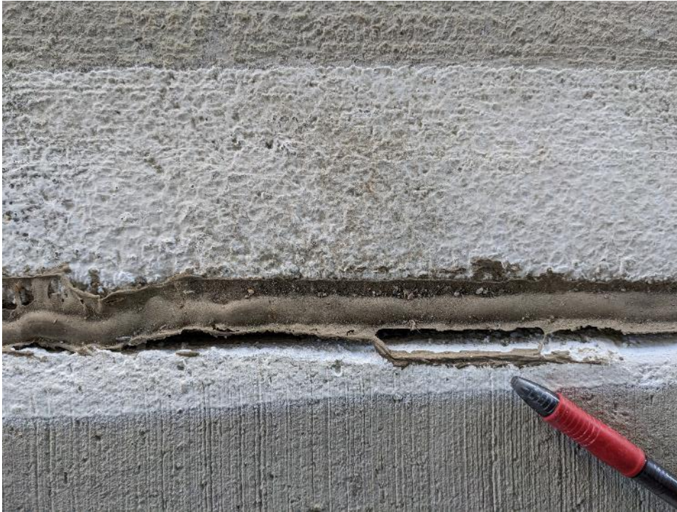
Photo 62. Cove sealant at the wall bases was typically missing at areas except at limited areas at the south end.
