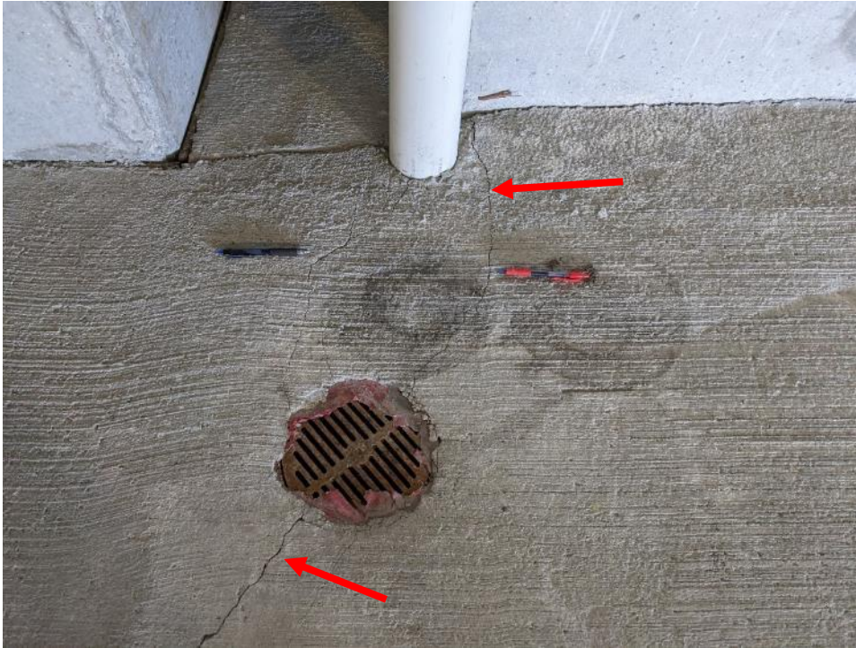
Photo 56. A wide crack that has stemmed off the corner of the column to the construction joint. Also note that the column perimeter is not sealed.
