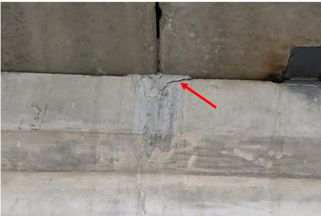
Photo 42. A small delamination of a beam haunch between hollow core planks along Grid Line 1.
