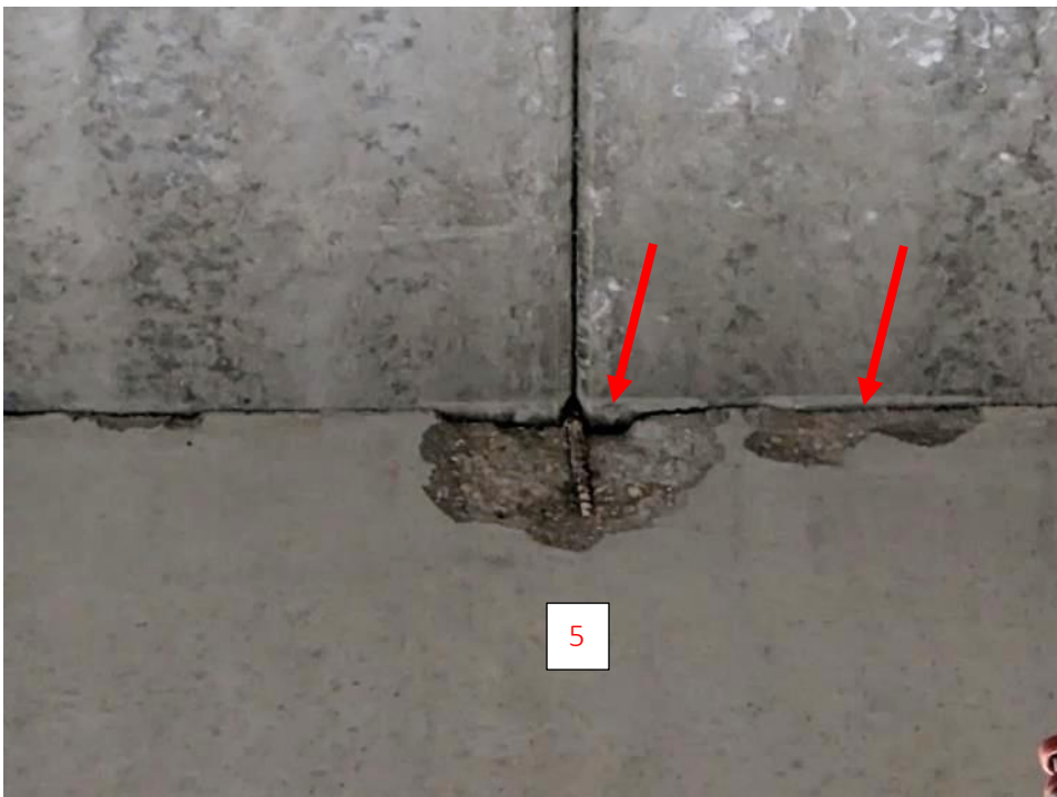
Photo 10. Spall 5 along Grid 7.8 from Photo 8. Note, presence of dowel at center of spall. Also note an adjacent small spall. Presence of a bearing pad is not obvious from ground.
