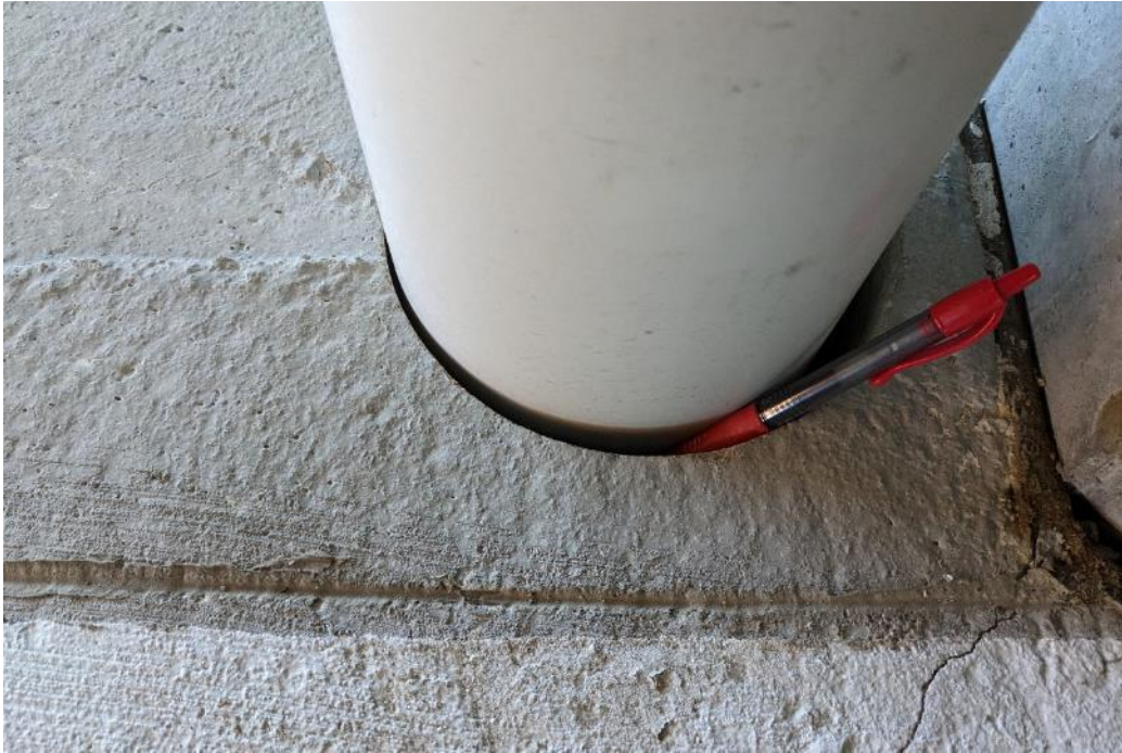
Photo 66. Pipe penetrations were typically not sealed. Also note floor crack extending from pipe penetration.
