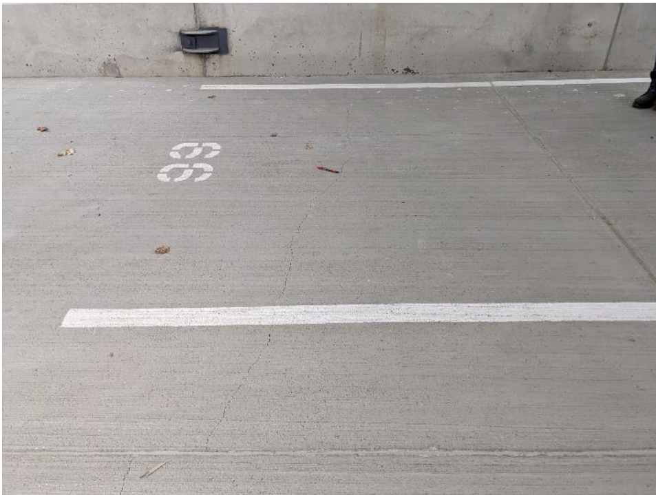
Photo 54. Typical crack in 2 nd level floor topping slab perpendicular to the hollow core planks.
