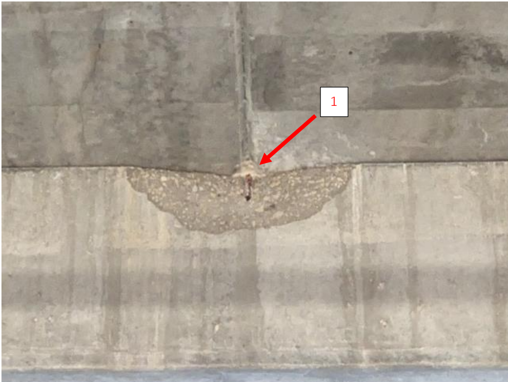
Photo 4. Close-up of the previous photo Spall 1. Note what appears to be a steel dowel with adhesive exposed at the center of the spall. Also note bearing pad is not present at edge.
