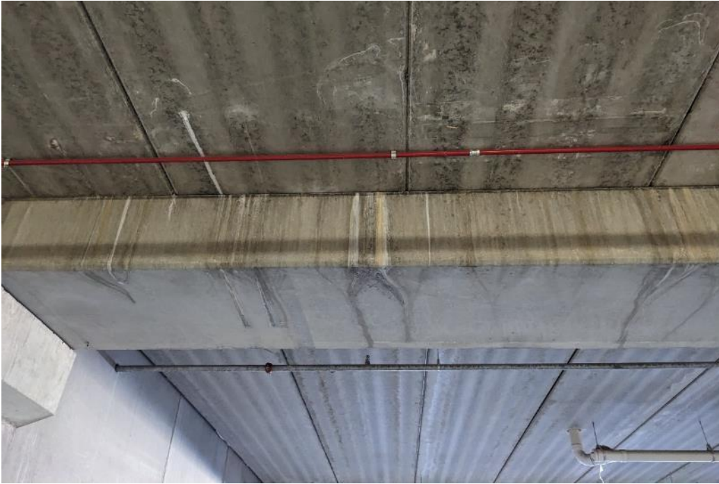
Photo 28. Water leaching and corrosion stains along the length of a beam observed from the 1 st level.
