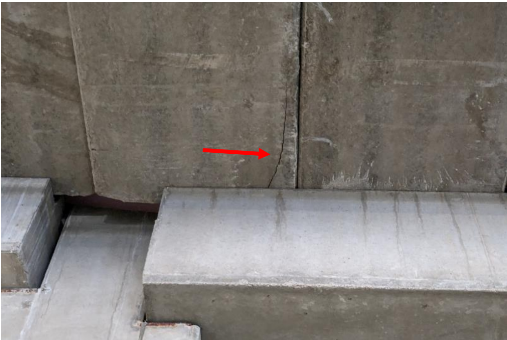
Photo 38. Close-up of the crack indicated in the previous photo.
