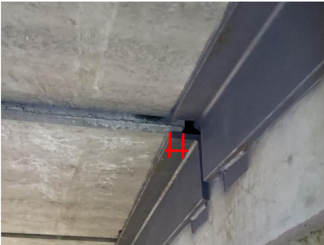
Photo 46. Minimal hollow core bearing at one location supporting the 2 nd level ramp.
