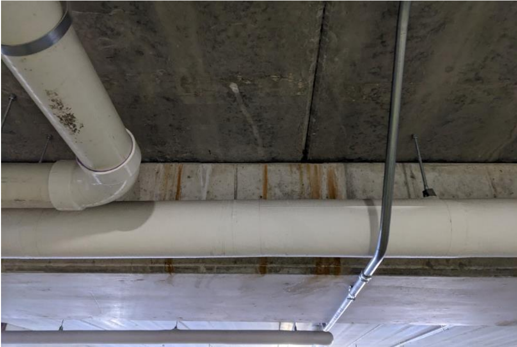
Photo 68. Corrosion staining along the length of a beam observed from the 2 nd floor.
