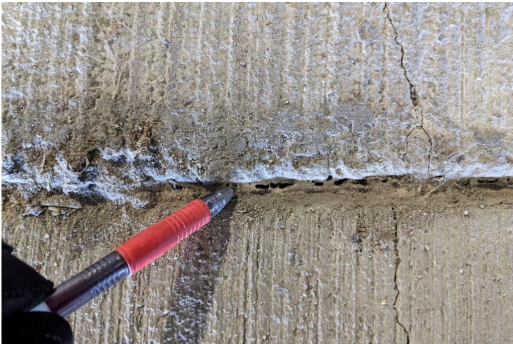
Photo 60. Additional failed construction joint sealant.
