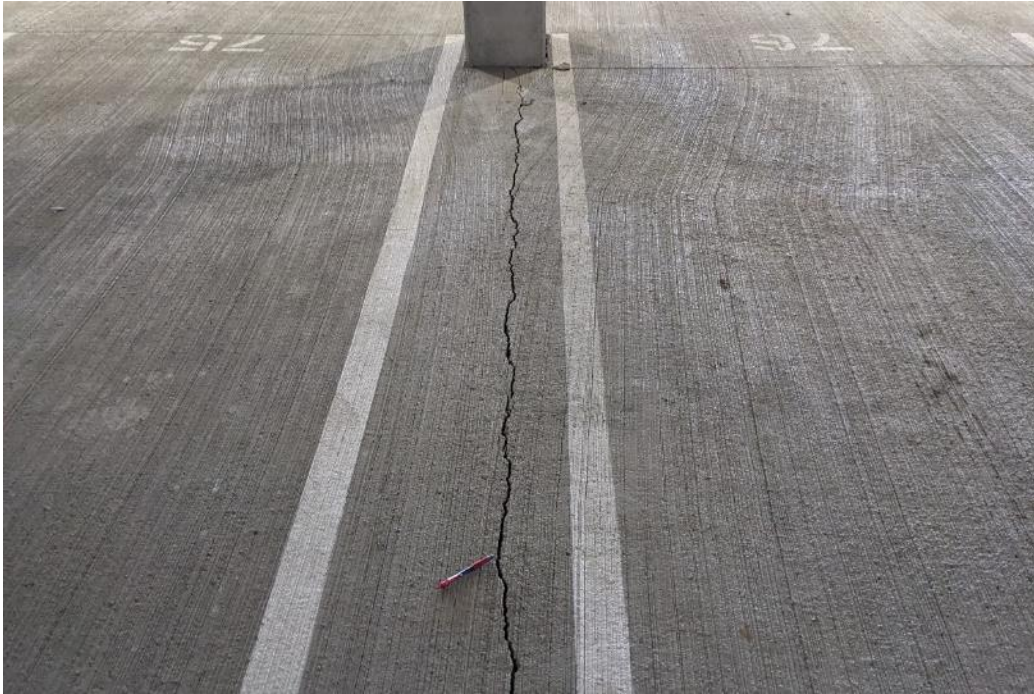
Photo 52. Small concrete spalls that have stemmed from the wide crack of the previous photo.
