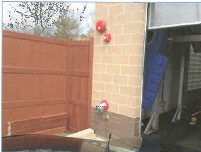
Figure 3 – A photo of the composite fence used in the Buffalo Grove facility.
