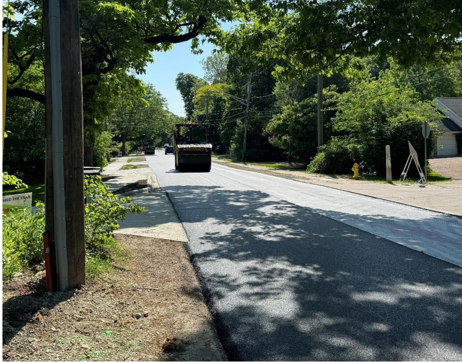
Hot-Mix Asphalt Surface Paving on Crescent Boulevard
