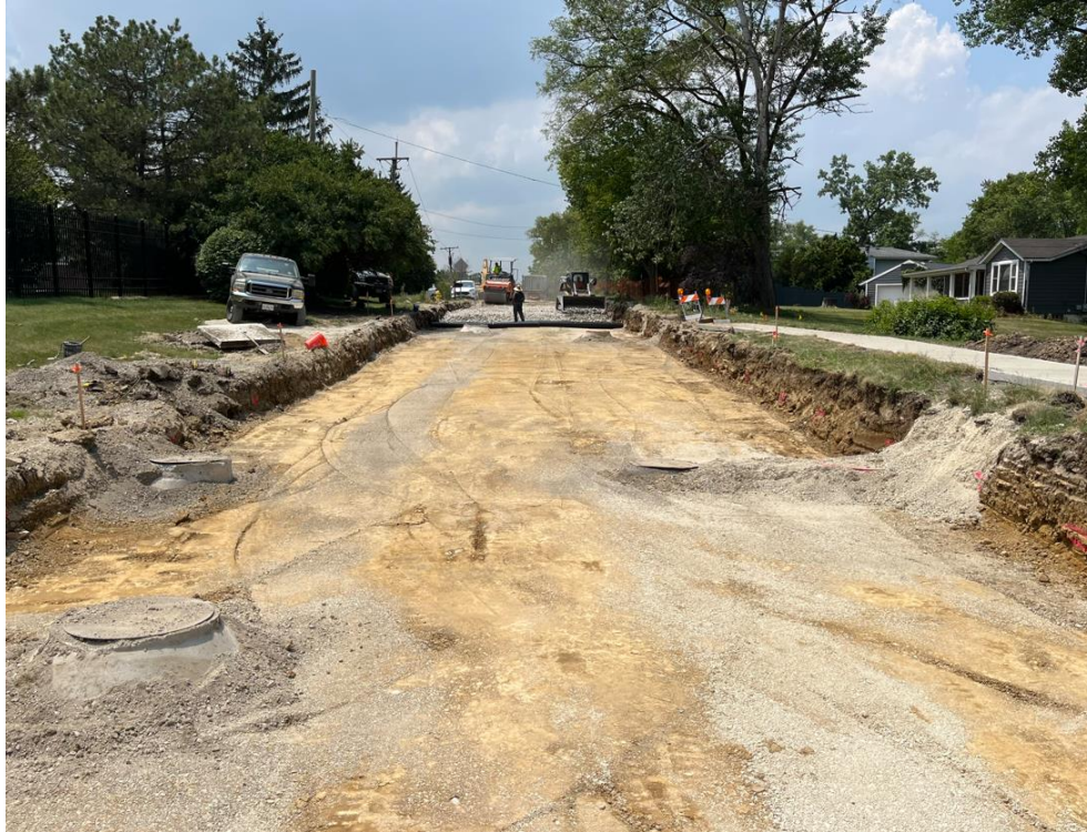
Roadway Excavation and Subgrade Construction on Bemis Road
