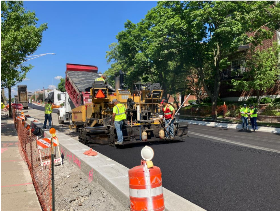
Asphalt binder being placed along Pennsylvania Ave east of Main Street
