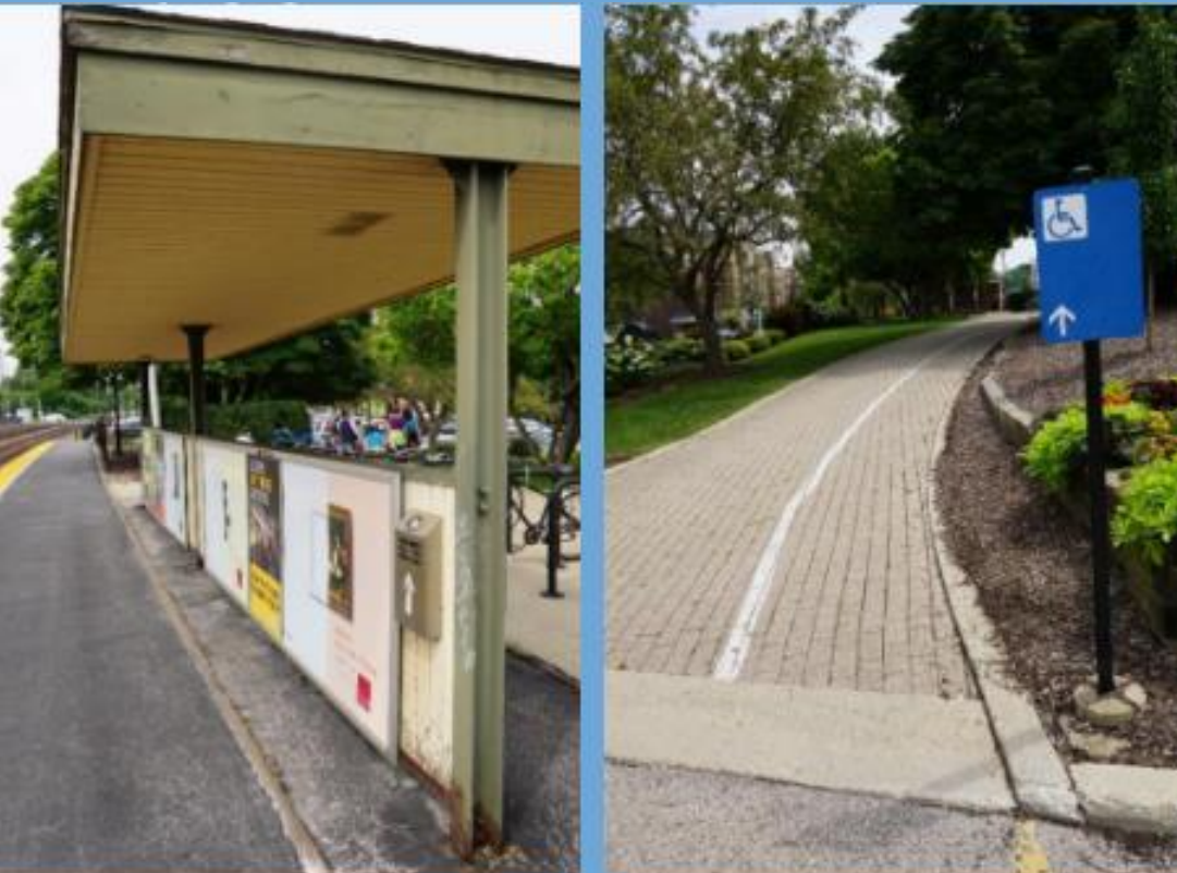
"Shelters" On Platform
