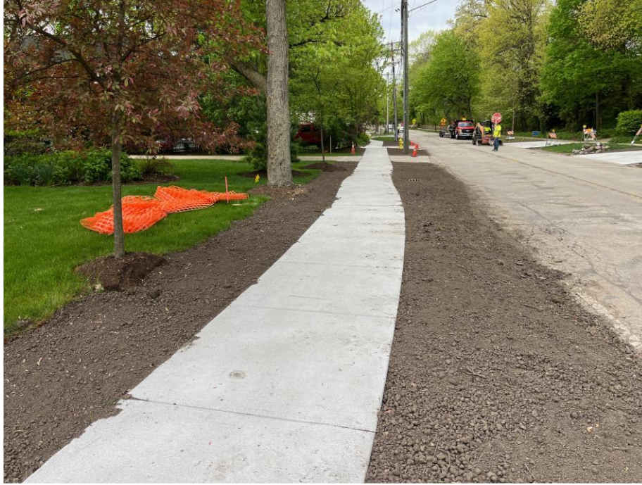
New sidewalk on Crescent between Lee and Riford.
