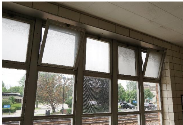
Figure 7: Existing aluminum single pane windows
