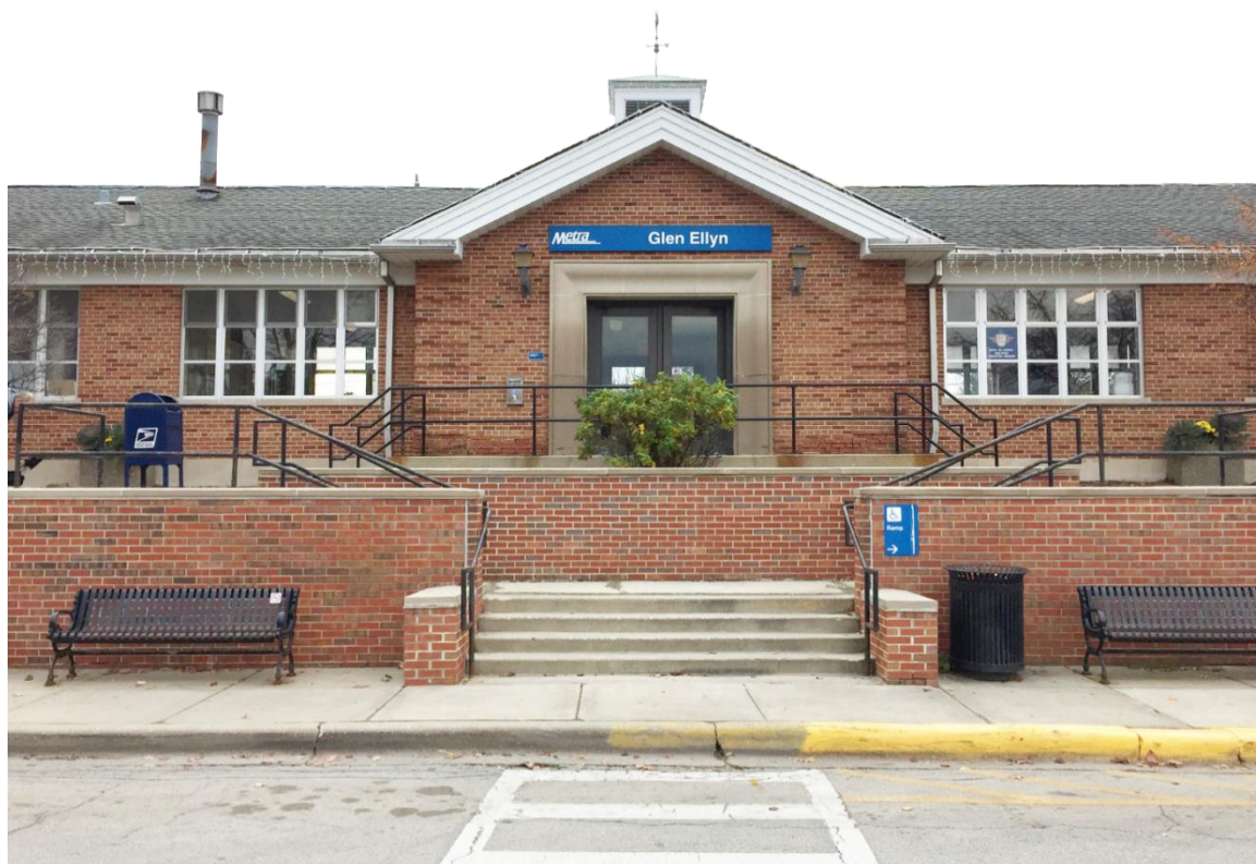
Figure 2-2 Existing Station Elevation from the North Looking South
