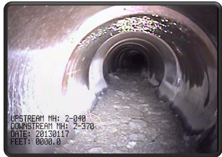
Sanitary Sewer Televising Video
