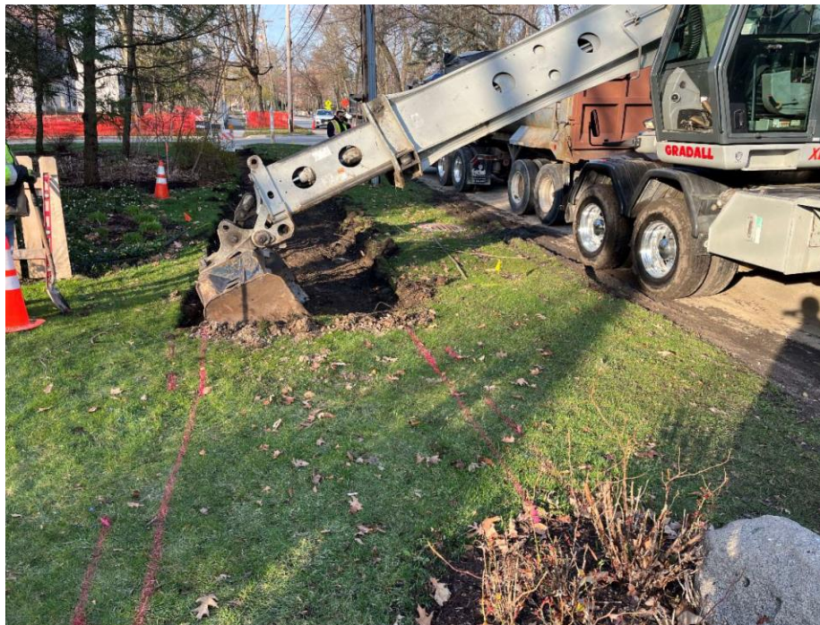
Excavation for new sidewalk between Lee and Riford.
