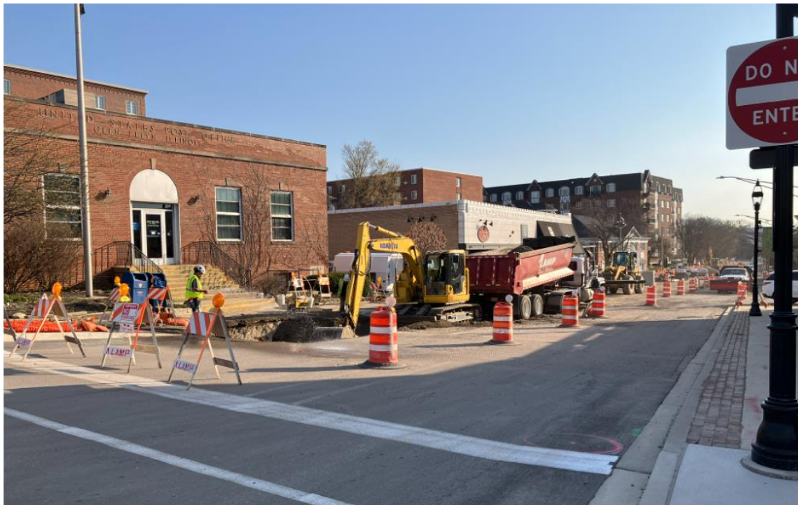
Start of installation of new watermain along Pennsylvania east of Main Street
