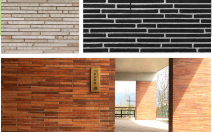
GLEN ELLYN AAC GUIDELINES Brick building facade
