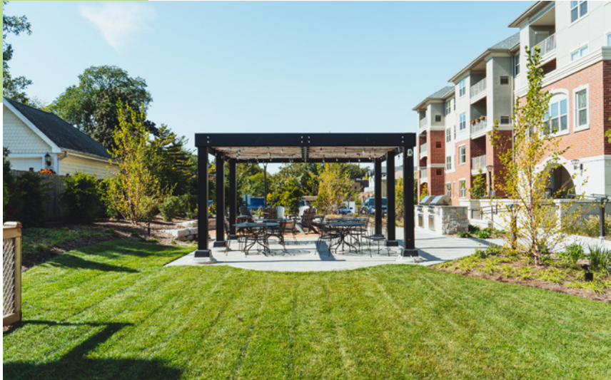
STEEL STRUCTURE Avere on Duane
