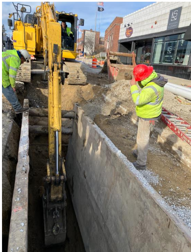
Installation of new sanitary sewer along Pennsylvania east of Main Street
