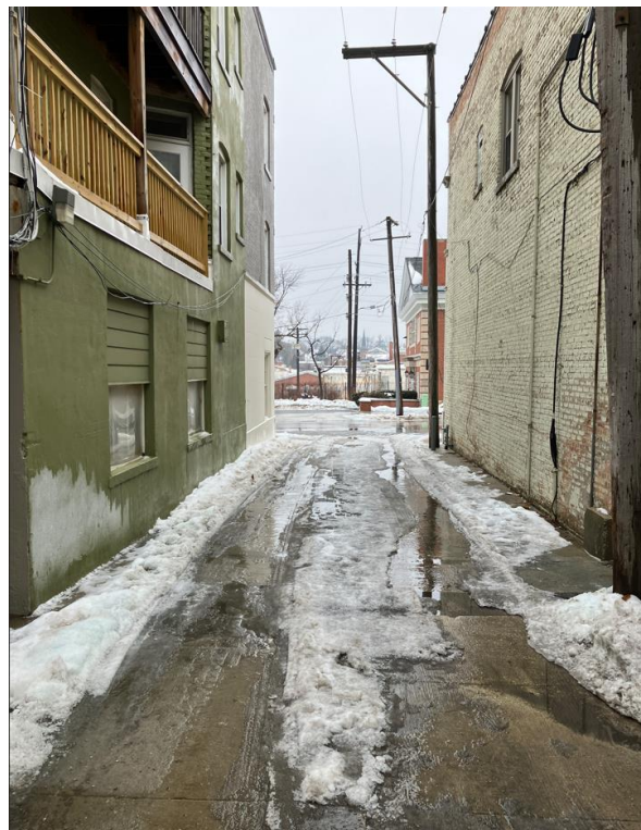
View from the alley looking north toward Duane Street. Coordination with ComEd has been conducted for bracing of the utility poles during underground utility excavation.
