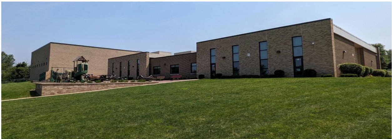
Current Churchill Elementary School Building, North Side
