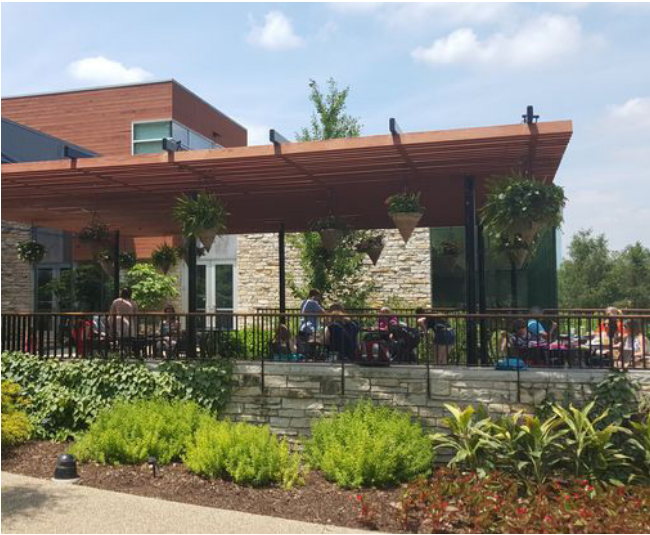
MORTON ARBORETUM Black steel structure with wood slats
