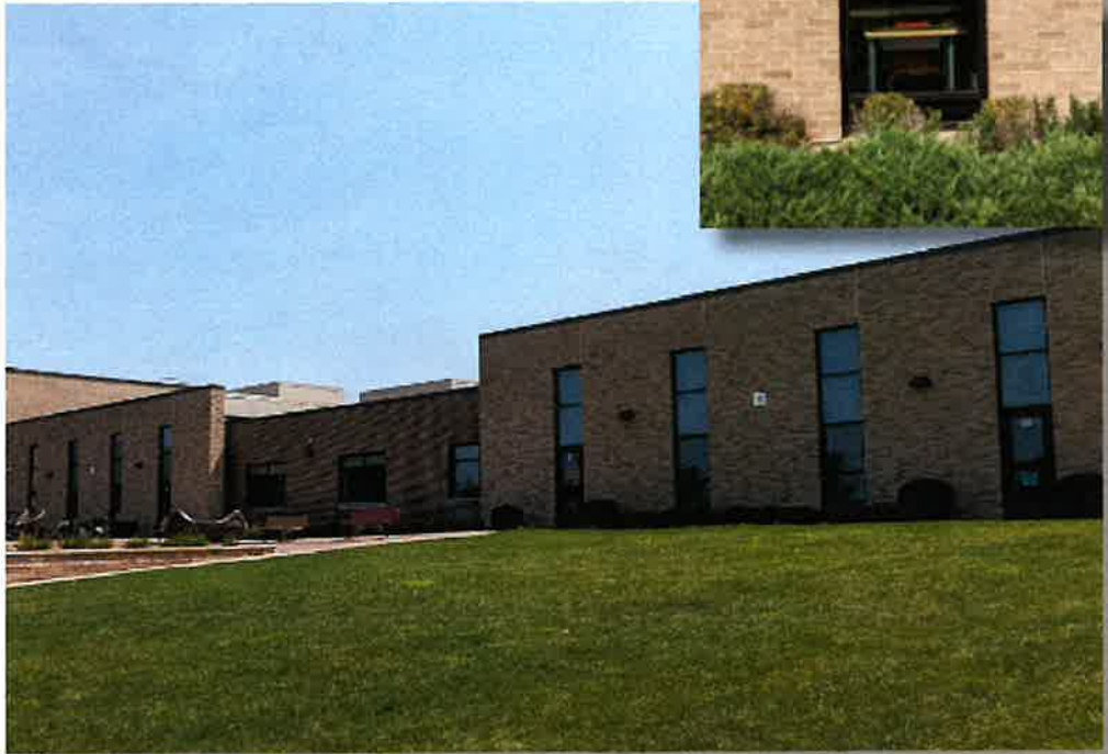
EXISTING ADJACENT BUILDING
