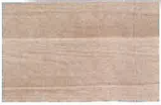
(H) POURED CONCRETE WITH FORMLINER
