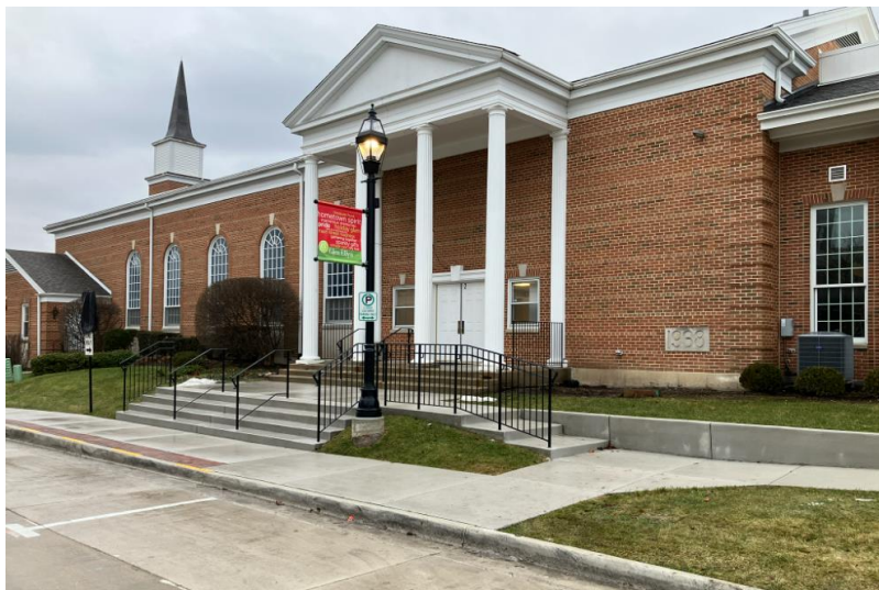
Newly-installed stairway railing within the public right-of-way at 501 Hillside Ave
