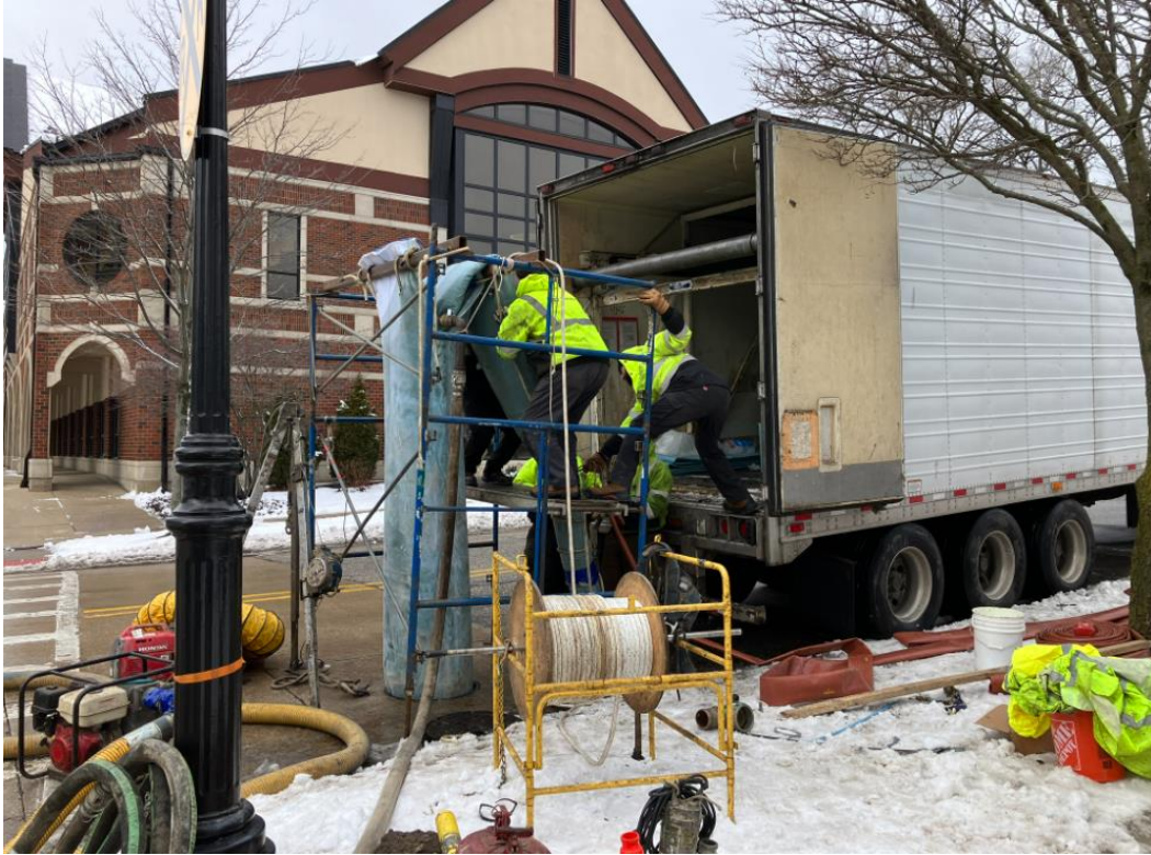
Storm Sewer lining along Prospect Avenue north of Duane Street
