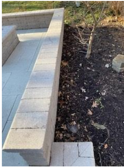
Seat wall on rear patio
