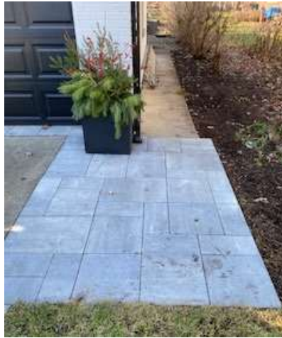
New paver additin to existing walkway
