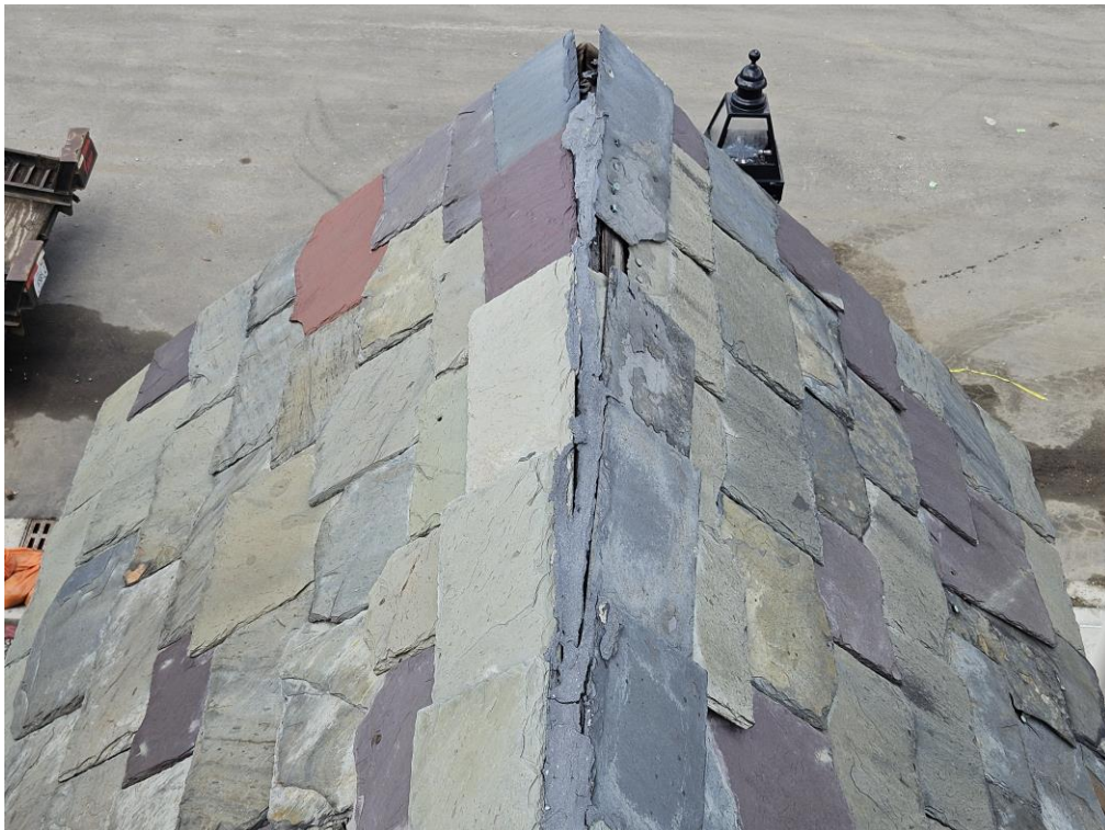
Images of existing roof condition
