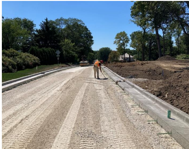
Preparation of Roadway Aggregate Subgrade Improvement on Hill Avenue – 9/1/2023
