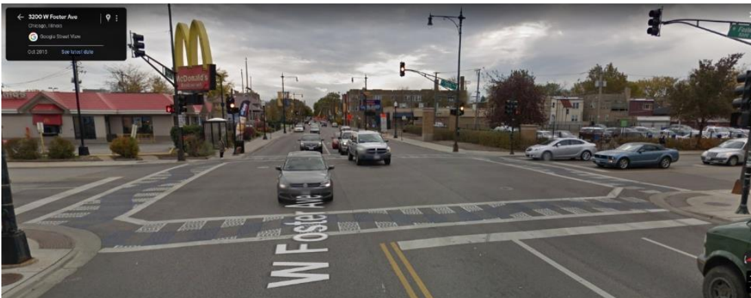
After image: Installed in 2015, note the more visible crosswalks with a pattern. Note this was reinstalled in 2021 because of pavement resurfacing. Photos are available to show the new appearance and the wear after one year. This pattern used inlaid thermoplastic so that snowplows did less damage to the pavement markings.
