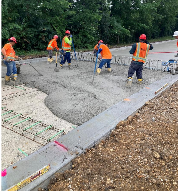
Hill Avenue Jointed Portland Cement Pavement Placement – 9/7/2023
