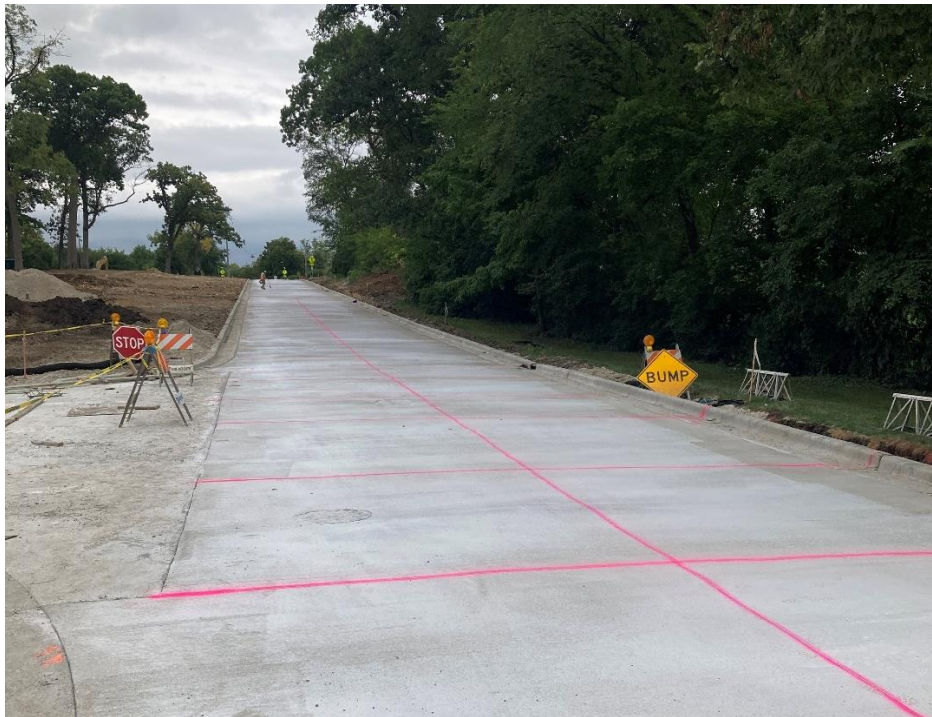
Layout of Hill Avenue Pavement Joint Sawcutting – Evening of 9/7/2023
