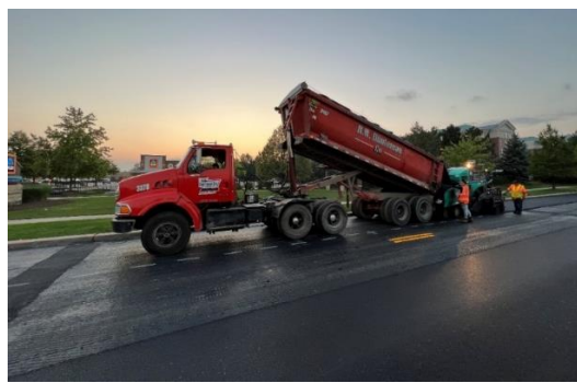
Repaving of the Nicoll Avenue Land Bridge (between Roosevelt Road and DuPage Boulevard) 8/29/2023
