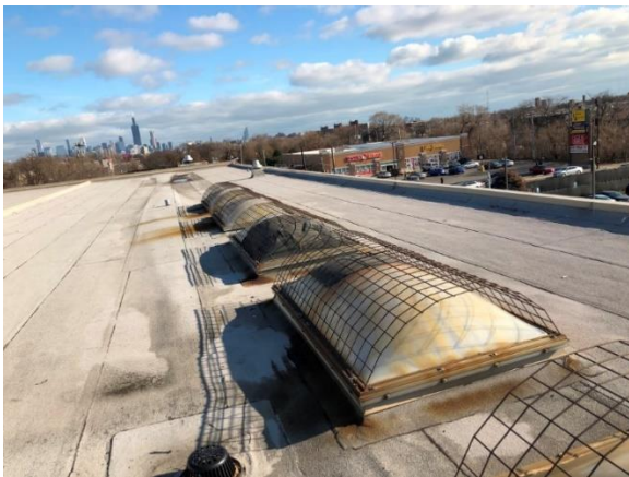
Example of Hail Damaged Skylight at the CTA Kedzie Bus Garage
