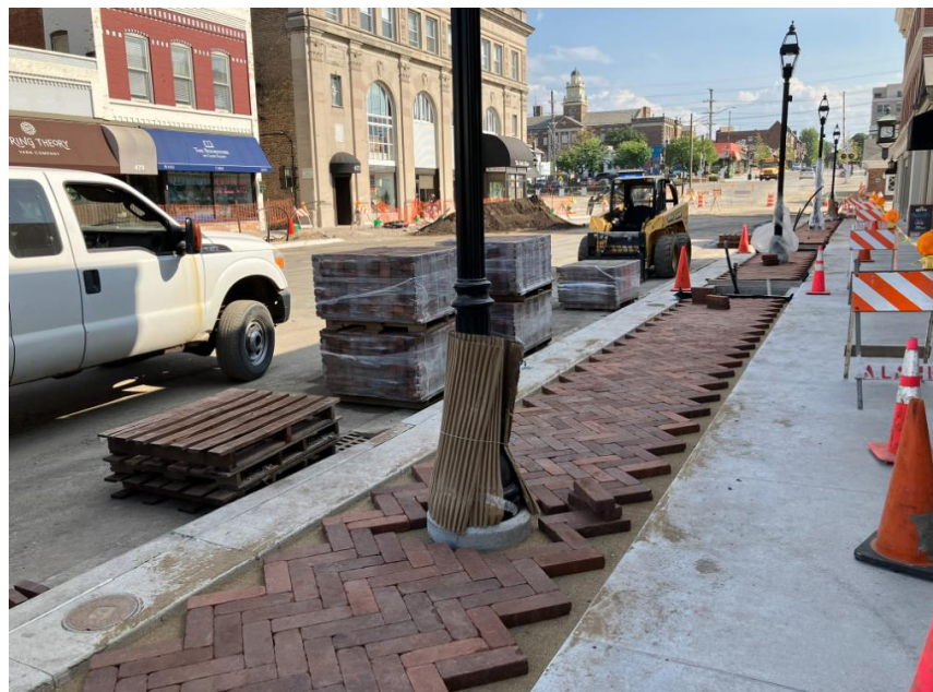
Brick pavers being installed along the west side of Main Street, south of Pennsylvania Avenue
