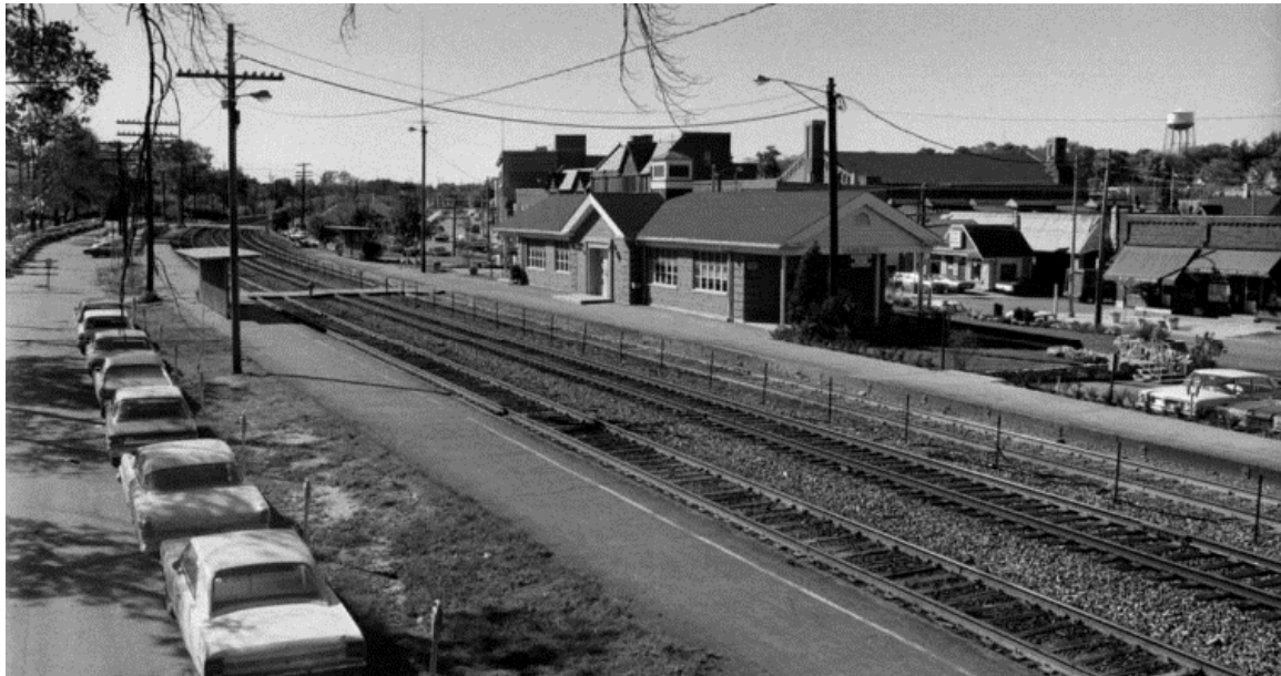
Existing Glen Ellyn Train Station, looking Northwest.
