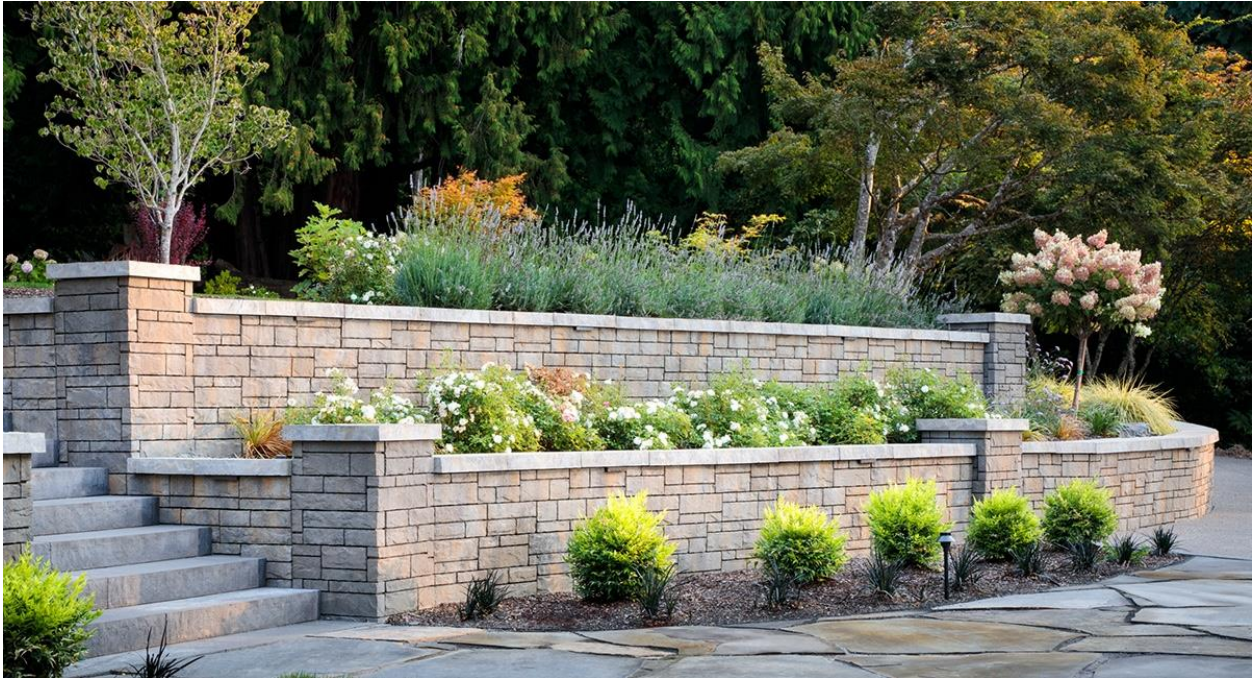
Modular block walls can include seat walls and can be adapted to various landscaping requirements.
