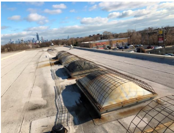
Example of Hail Damaged Skylight at the CTA Kedzie Bus Garage
