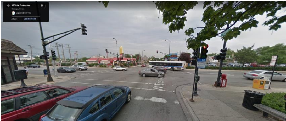
Before image: Note the crosswalks are barely visible and worn. Little conveyance to drivers that this intersection is also used by pedestrians.
