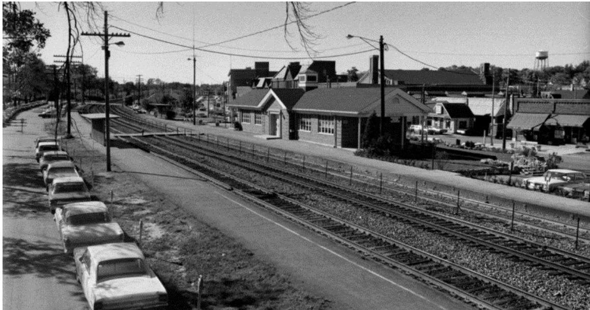
Existing Glen Ellyn Train Station, looking Northwest.
