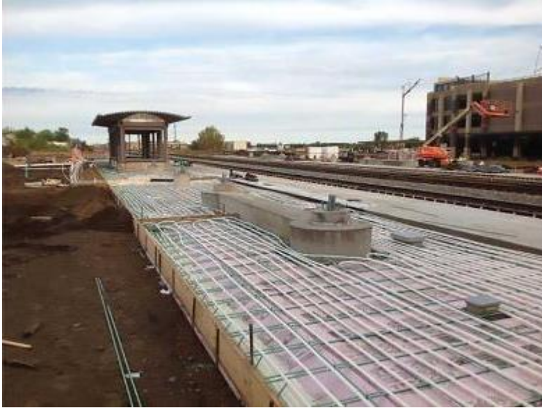
Heated Railway Platforms tested to avoid ice accident (Minnesota case study)
