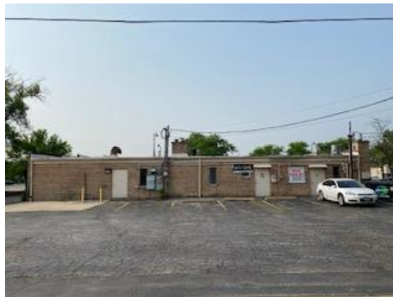
Rear (North) Elevation along alley.
