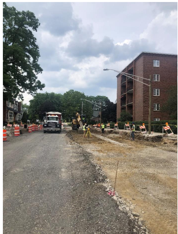
Roadway Excavation and Subgrade Improvement Construction along Main Street between Anthony and Pennsylvania
