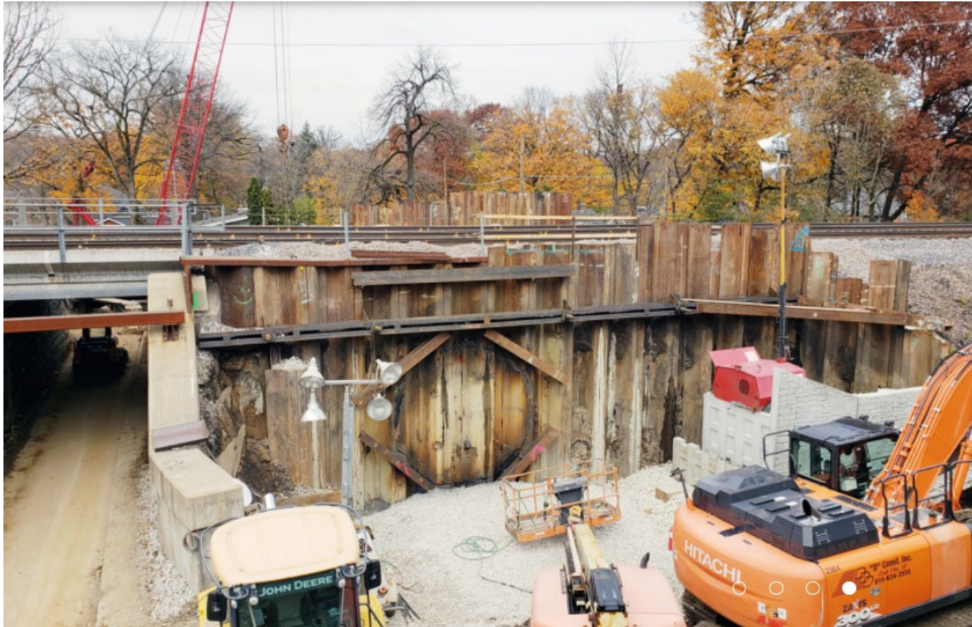
Preparation of the “push pit”
