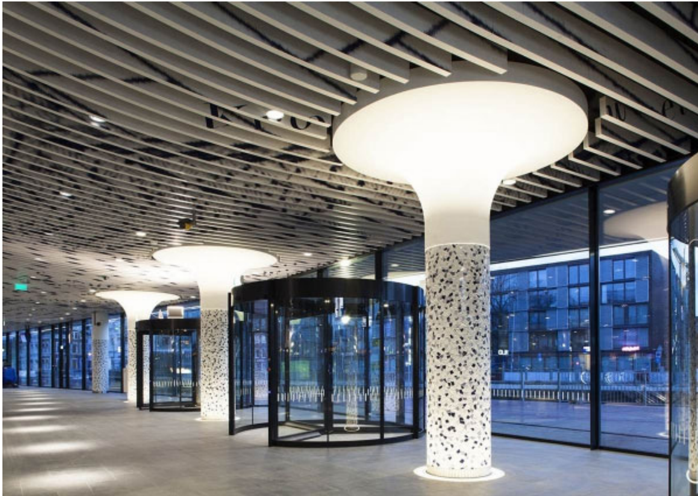
Structural Columns inside Delft Train Station, Netherlands
