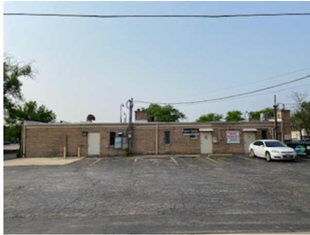
Rear (North) Elevation along alley.
