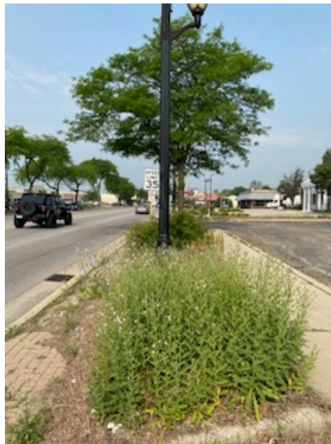
Existing condition of Roosevelt Road parkway.
