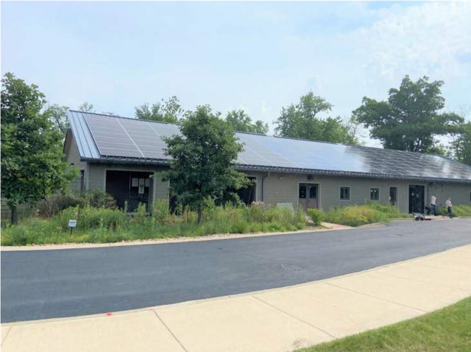
PHOTO 2 - EXISTING SPECIES PROPAGATION BUILDING
