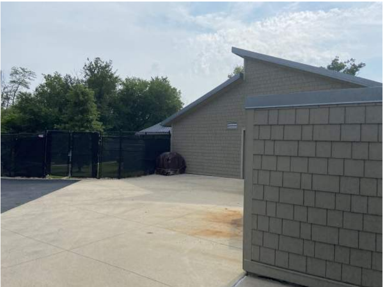
EXISTING PROPAGATION BUILDING
