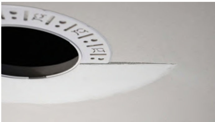
Partially finished mud ring, showing cross-section detail.
